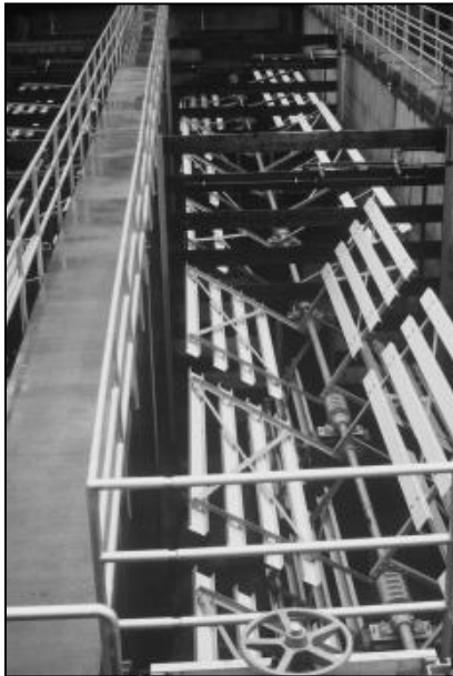
Figure 3-5 Paddle wheel flocculator, with three stages of energy input achieved by decreasing paddle area for each stage
