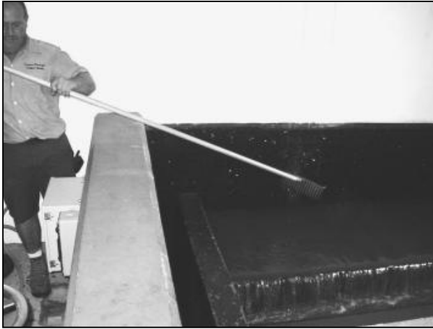
Figure 10-17 Mudball rake to remove mudballs from a small filter
