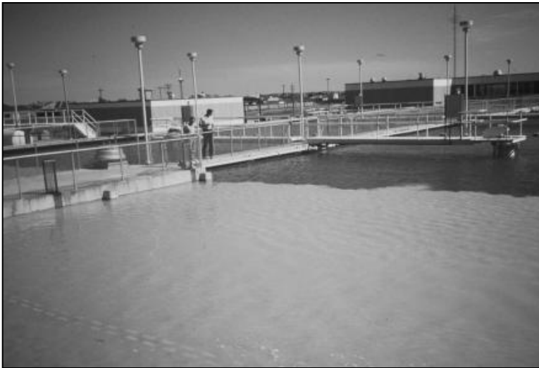
Figure 2-1 Dramatic improvement in clarity at lime softening plant as water enters sedimentation basin
