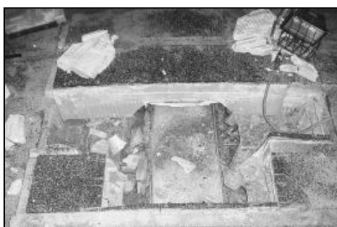
Figure 10-3 Uplift failure of filter underdrain tile system with porous plate cap
