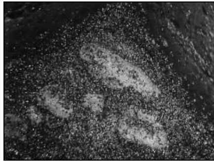
Figure 6-2 Mudballs on top of filter bed
