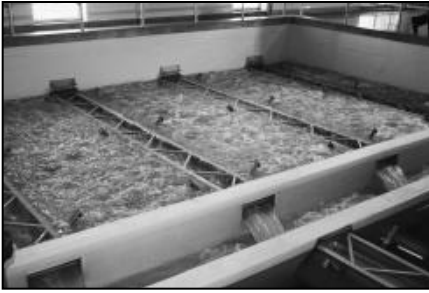
Figure 6-5 Filter backwash with uniform air scour
