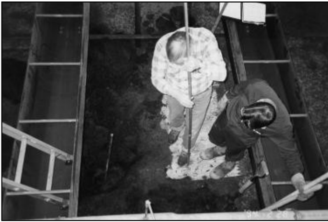
Figure 10-8 Probing filter media to locate large lumps of material in bed
