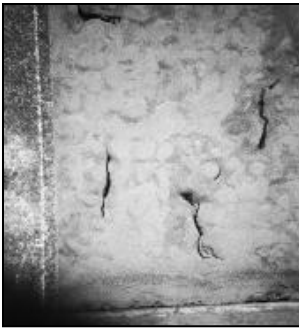
Figure 6-1 Cracks in filter bed
