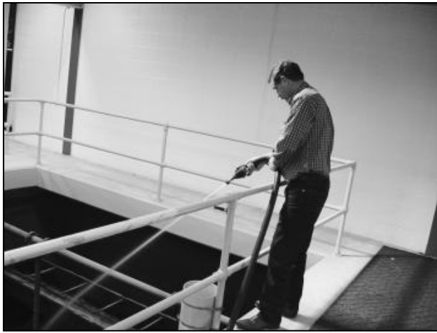
Figure 10-19 Hosing a filter to break up mudballs
