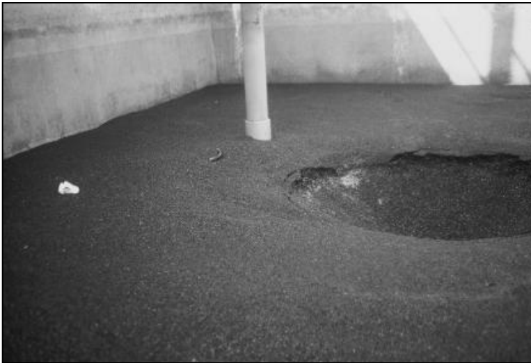
Figure 6-10 Cone of depression in filter media resulting from loss of nozzle in filter bottom
