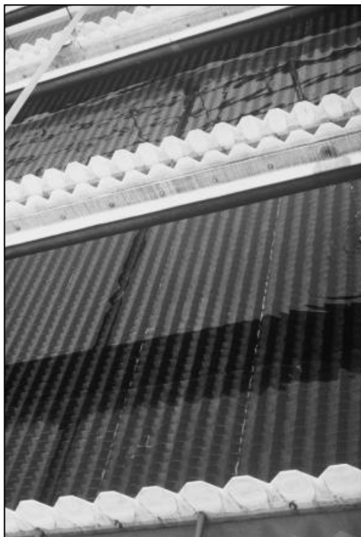
Figure 3-11 Tube settlers in settling basin producing very clear effluent
