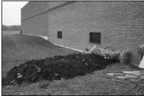
Figure 10-5 Filter media removed from pressure filter shown in Figure 10-4
