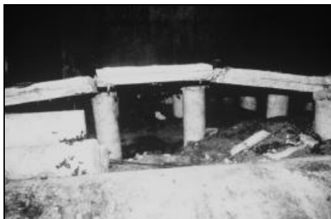
Figure 10-1 Uplift failure of false floor in filter
