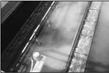
Figure 6-5 Filter backwash with uniform air scour
