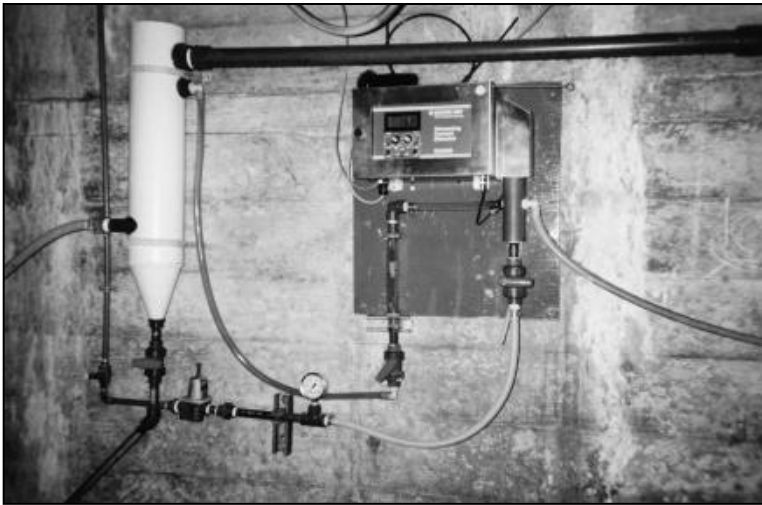
Figure 2-5 Streaming current instrument installed at water treatment plant
