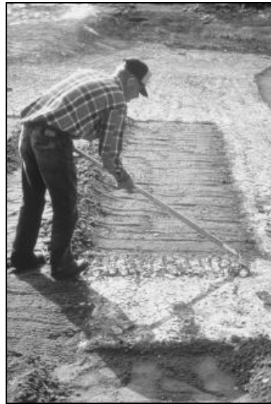
Figure 11-8 Manual cleaning of a slow sand filter
