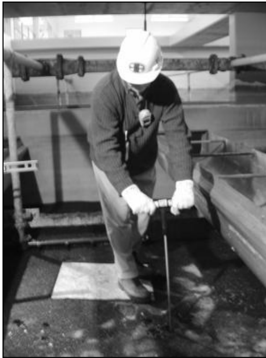
Figure 10-7 Probing to determine depth of filter media to support gravel
