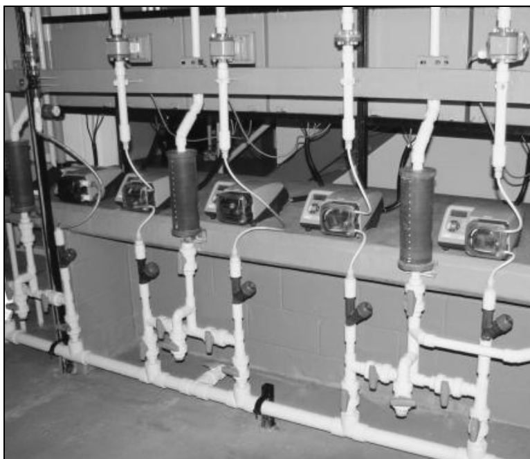
Figure 9-3 Chemical feed pump calibration apparatus
