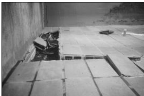
Figure 10-2 Clay tile filter underdrain failure
