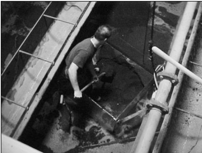
Figure 10-11 Digging media out of excavation box
