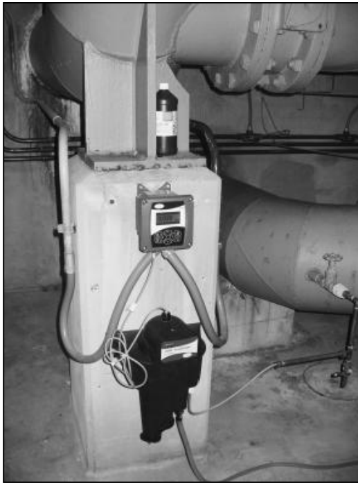
Figure 9-2 Turbidimeter mounted in pipe gallery
