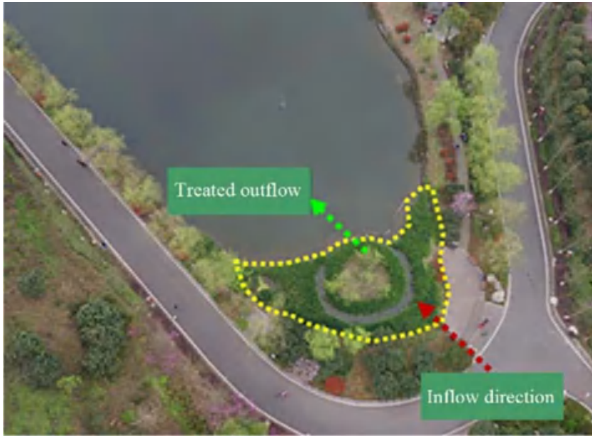
Figure 13.13 Aerial view of enhanced lateral-flow biological filter for lake inflow quality control (photo by authors).
