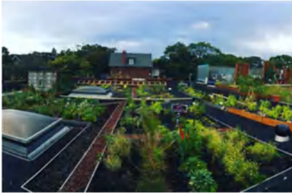
Figure 4.9 Example of a green roof (source: greenroofs.org).
