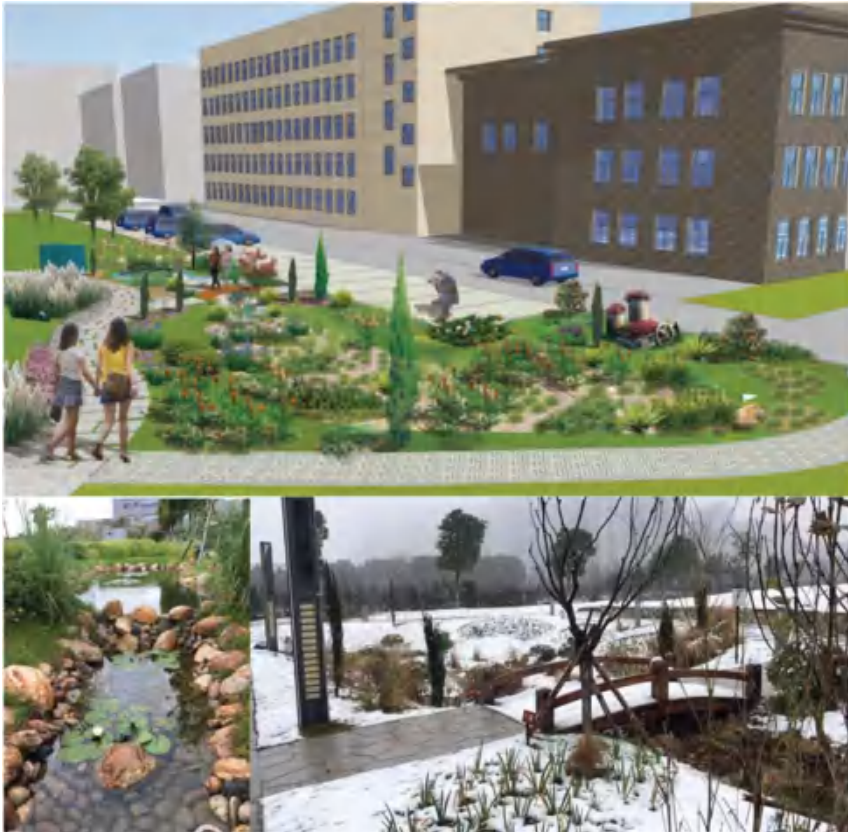
Figure 5.5 Landscape design concept (top), the recreational pond (waterscape) that receives treated stormwater (bottom left), Arch timber bridge between the pond and biofilter (bottom right, in winter).
