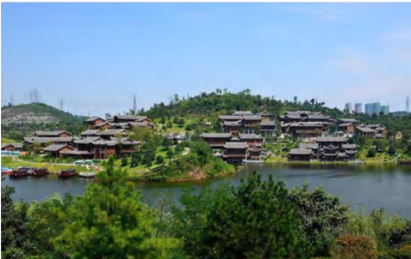
Figure 13.17 Real scene of part of the Longjing Lake surrounded by restored traditional houses (photo by authors).
