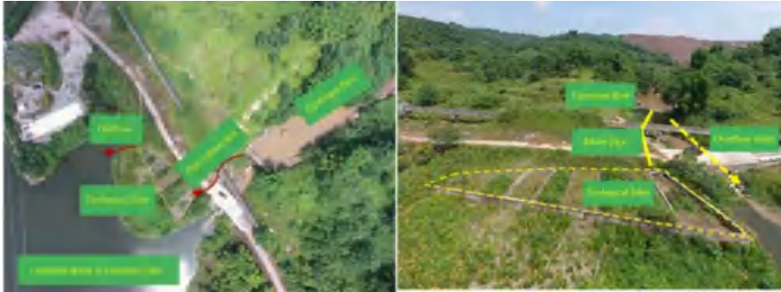
Figure 13.11 Location of ecological filters in the Zhaojia River Ecological Park (photos by authors).
