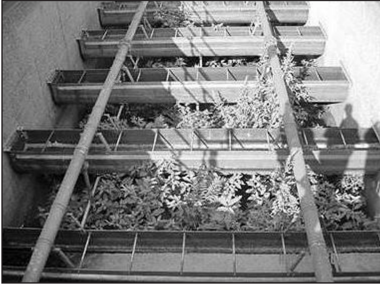
Figure 15-1 An out-of-service filter in an active plant
