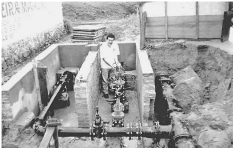
FIGURE 18.29 Valve being installed on bypass, contract No.3.066/98.
