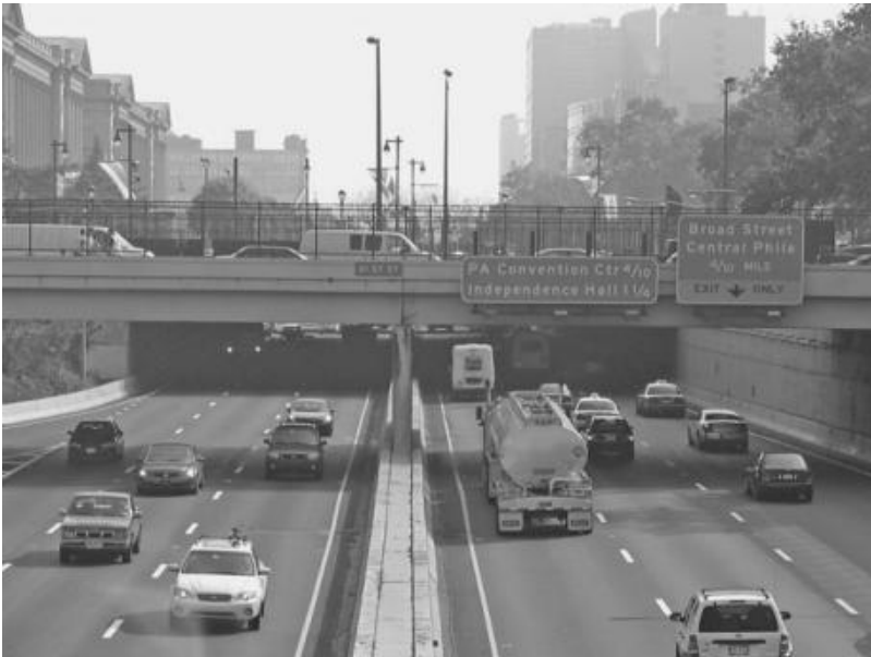
FIGURE A.1.7 Bridge over interstate highway in Philadelphia; leaks exist on 48-in steel main traversing under this highway. (Source: Philadelphia Water Department.)
