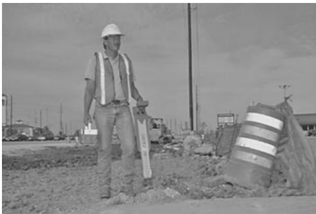
FIGURE 16.5A Using a pipe locator.
