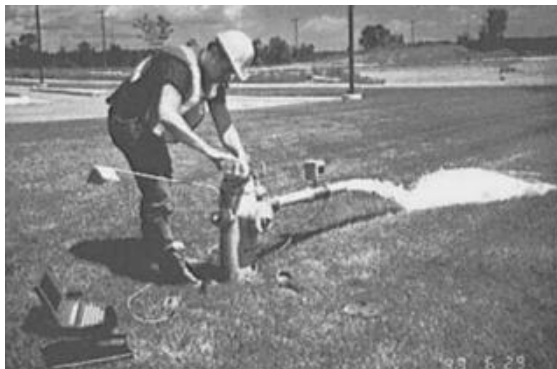
FIGURE B.18 Turbine hydrant meter. (Source: Julian Thornton.)
