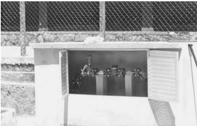
FIGURE 18.30 Above ground assembly, contract No.3.066/98.
