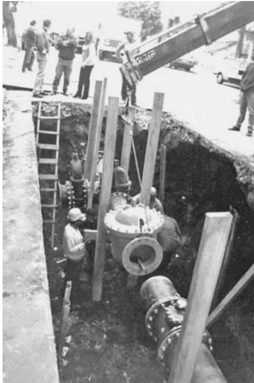
FIGURE 18.28 Valve being installed on main line, contract No.69.502/96.
