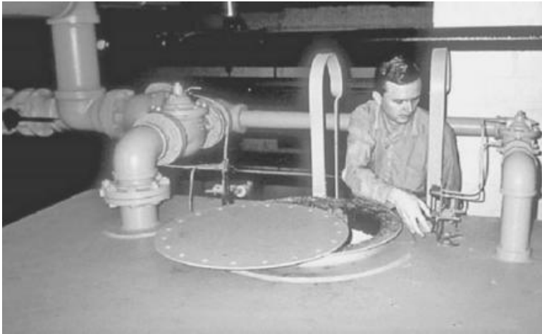
FIGURE 18.16 Calibrating a ball valve.
