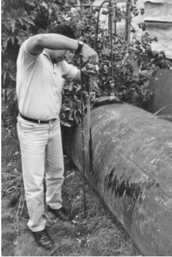
FIGURE B.1 Pitot rod installation. (Source: BBL Ltda.)
