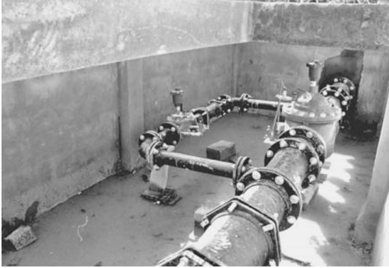
FIGURE 18.23 Parallel installation unequal diameters, contract No.3.066/98.
