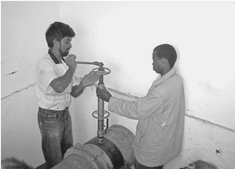
FIGURE B.7 Under pressure tapping. (Source: Restor Ltda.)
