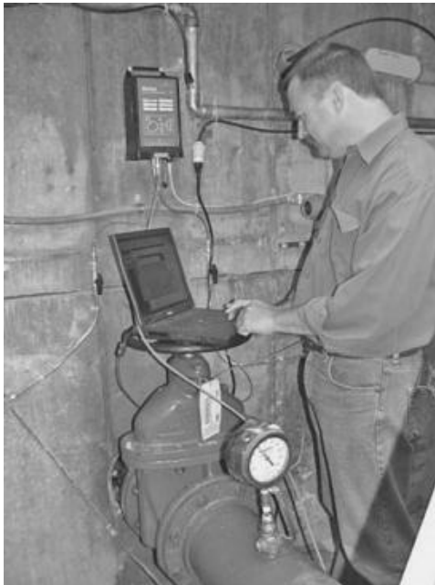
FIGURE A.1.3 The author, Julian Thornton, performs startup calibration of the electronic controller for Philadelphia's DMA5. (Source: Philadelphia Water Department.)
