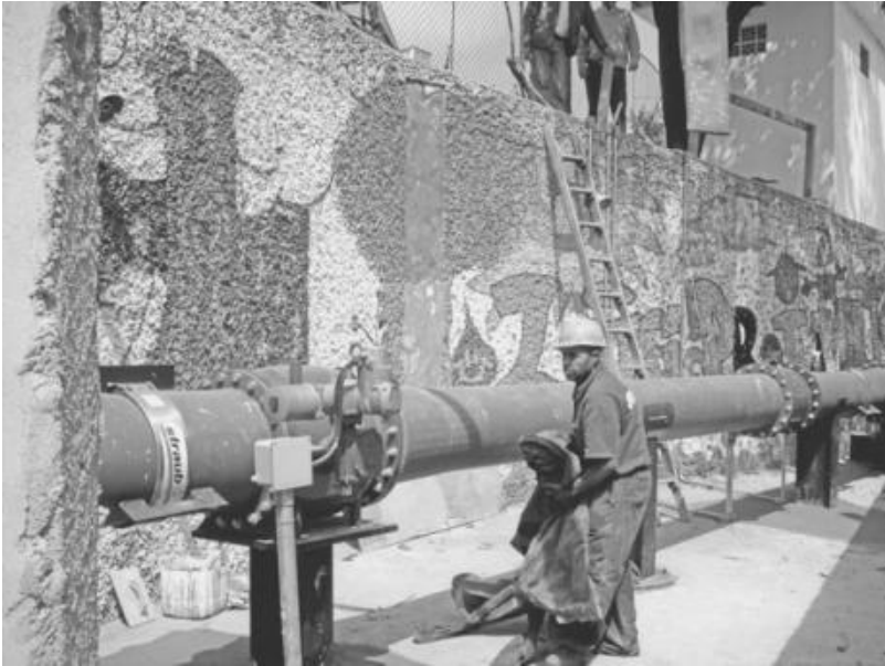
FIGURE 18.33 Plunger valve installation in Sao Paulo SABESP MS.
