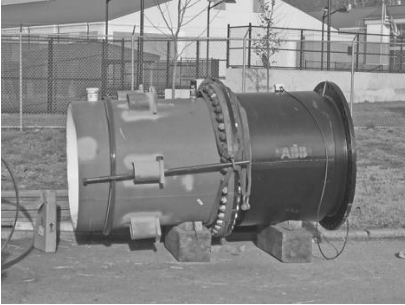
FIGURE 6.3 Source meter replacement at raw water pumping station: New 48-in diameter magnetic meter being prepared for installation. (Source: Philadelphia Water Department.)
