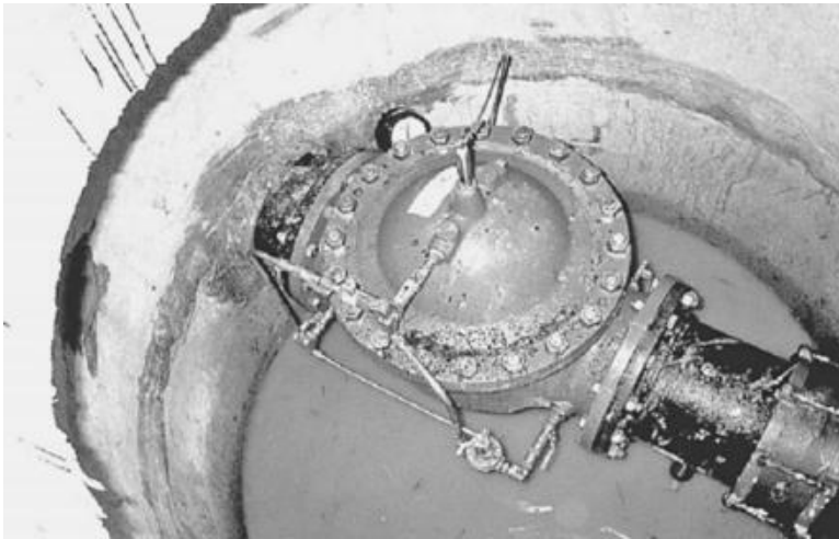
FIGURE 18.20 Sustaining valve installation.
