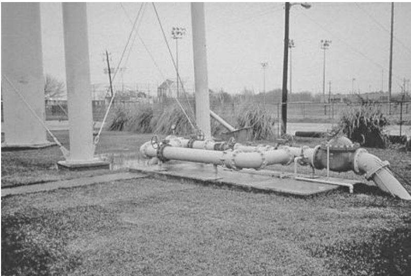
FIGURE 22.9 Altitude valve. (Source: Watts ACV, Houston, Texas.)
