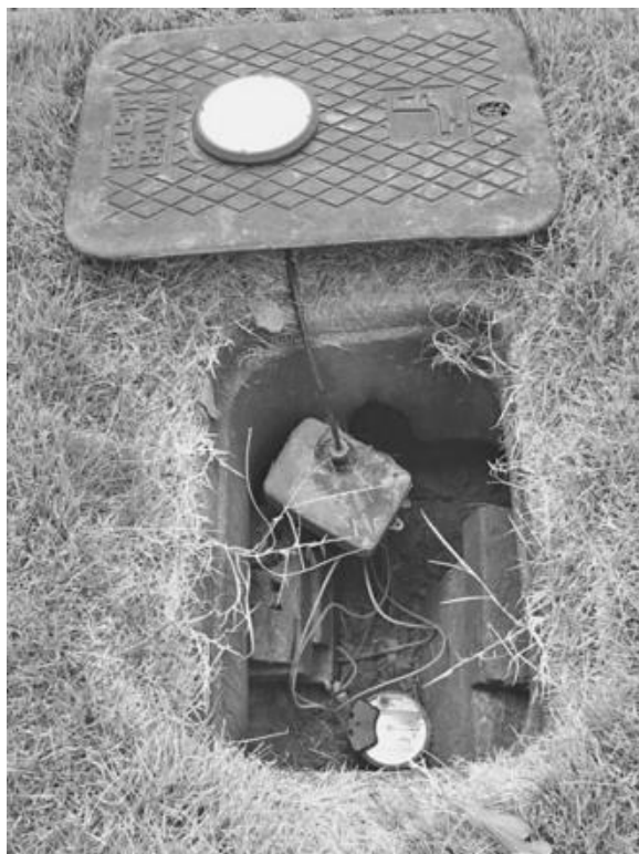
FIGURE 13.3 Typical outdoor meter pit installation. (Source: Neptune Technology Group.)
