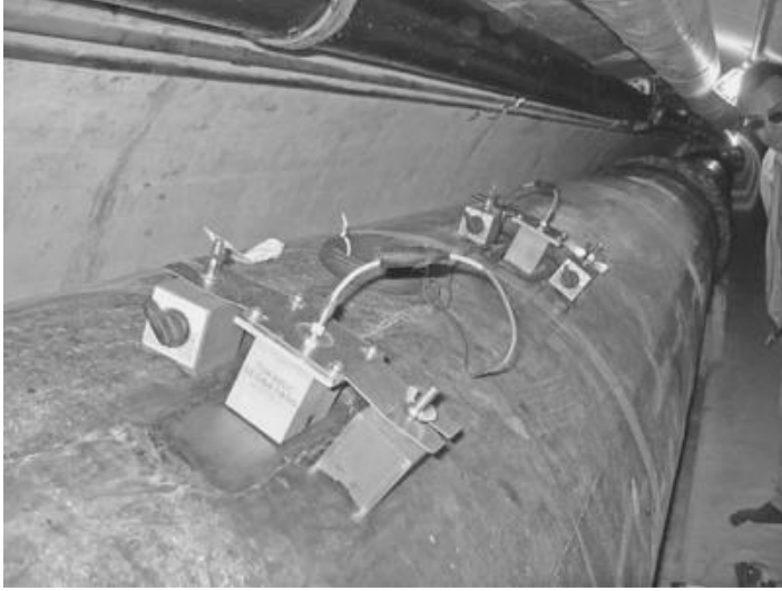
FIGURE B.16 Clamp on ultrasonic meter. (Source: Reinhard Sturm.)
