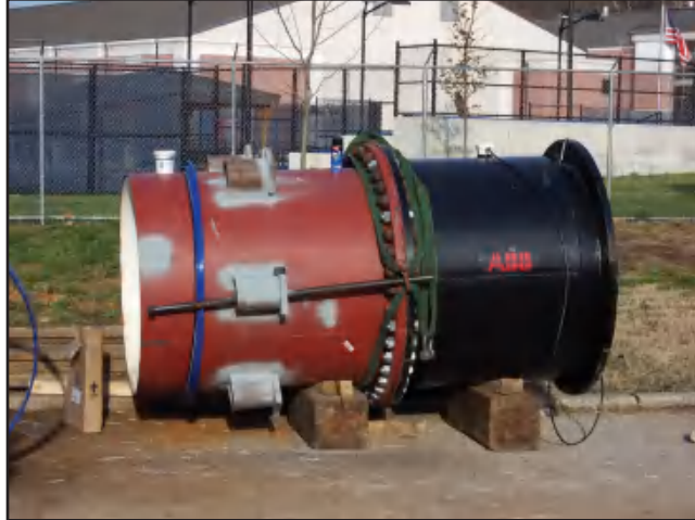
Figure A-1 Magnetic flowmeter awaiting installation on a 60-in.-diameter raw water pipeline in Philadelphia, Pa.
