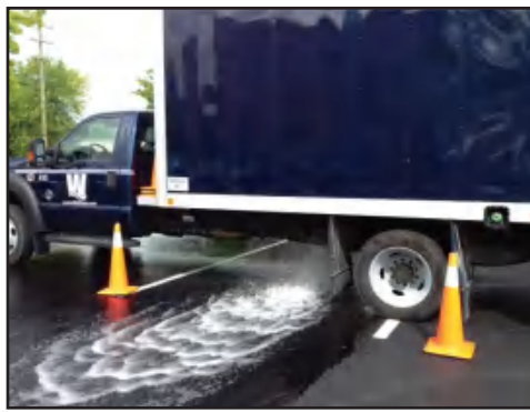
Figure 5-13 Water being discharged to waste during large meter testing operation. Utilities should be certain to follow applicable state and local requirements for the safe discharge of drinking water to surfaces.
