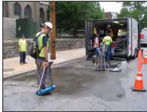
Figure 7-22 Use of inline leak detection technology in a 48-in. water main
