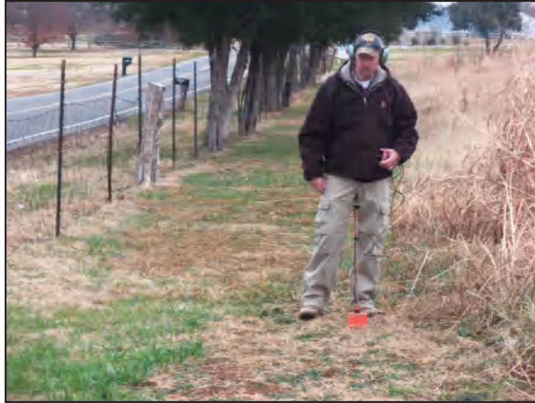
Figure 9-1 Using a ground microphone to listen for leak noise on piping in an unpaved surface in Wilson County, Tenn.
