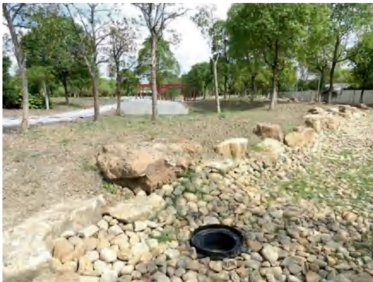
Fig. 5 Rain garden under construction in the first round Sponge City Jiaxing (September 2016)
