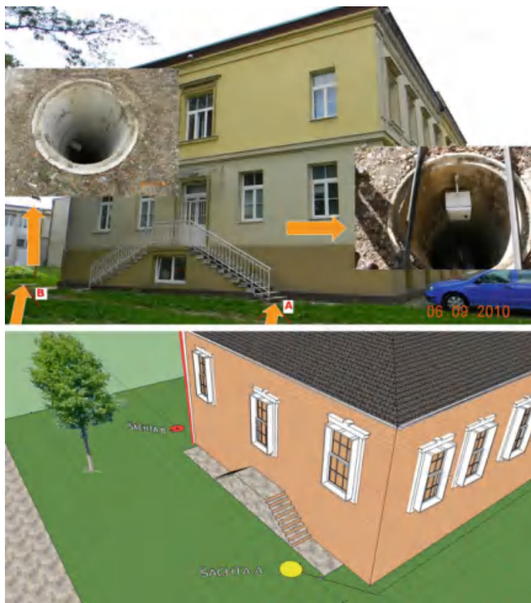
Fig. 19 Location of infiltration shafts near building PK6 (Markovič and Vranayová 2013)
