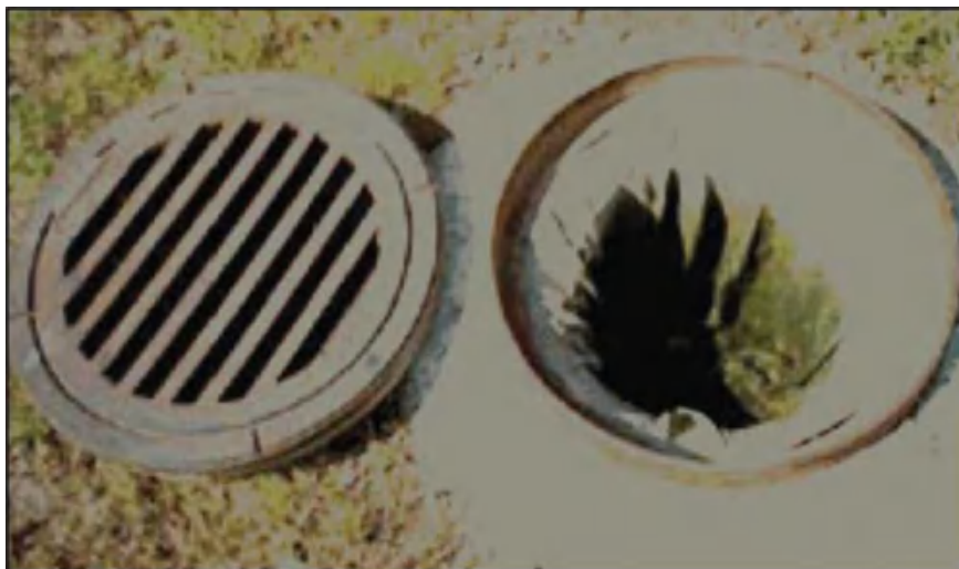
Fig. 5 Spillway shaft with a filter bag
