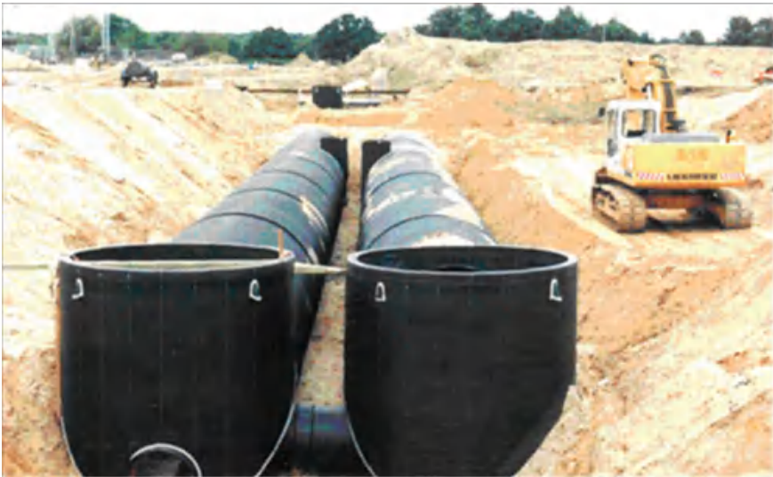
Fig. 10 Example pipe retention tank construction
