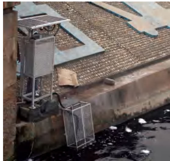
Figure 6.2: Riverside monitoring station.
