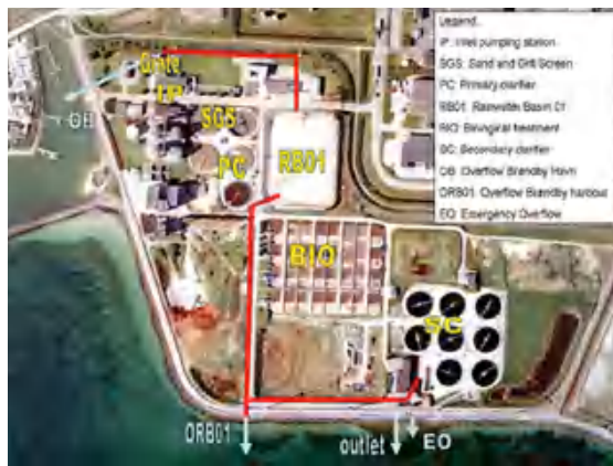
Figure 6.24: Aerial view of Avedøre WWTP.
