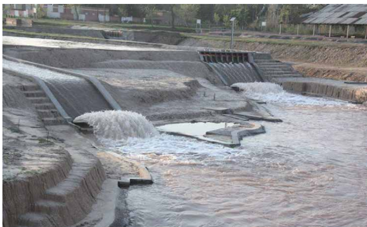
Figure 1. Flow from Flip Bucket Energy Dissipater.
