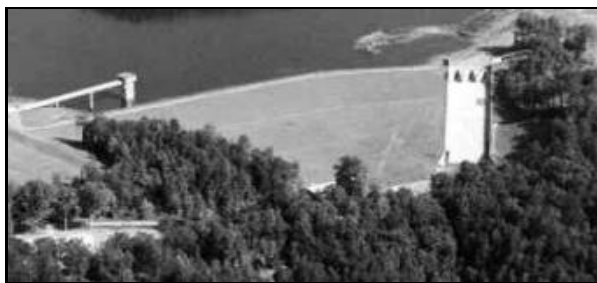
FIGURE 3-5 Yellow Creek Dam. Intake structure is to the left of the dam, and chute spillway is to the right of the dam.
