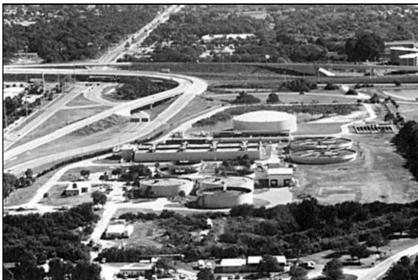
FIGURE 4-6 Reclamation plant in St. Petersburg, Fla., that incorporates secondary treatment, filtration, and chlorination
