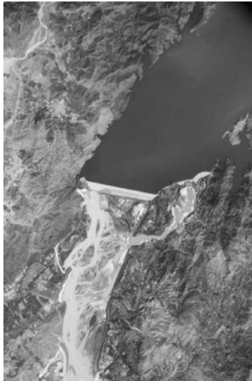
Satellite image of Tarbela Dam on the Indus River in Pakistan (Courtesy, Johnson Space Center, NASA)
