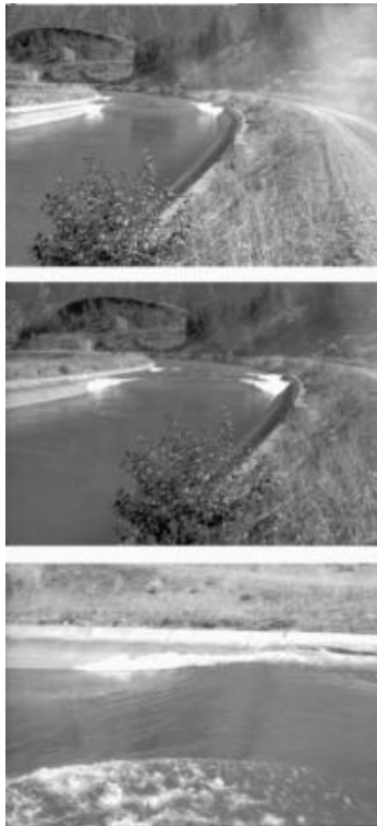
Propagation of surge wave in Seton Canal produced by the closure of turbine gates at the downstream end (Courtesy, British Columbia Hydro and Power Authority, Canada)
