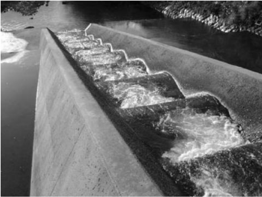
Flow conditions in a trapezoidal fishway, Japan (Courtesy, Prof. Y. Yasuda)
