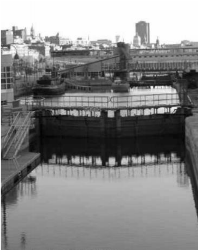
Lachine canal in Montreal, Canada, built during 1821 for shipping navigation, is 13 km long and 5.5 m deep (Courtesy, Prof. H. Chanson)
