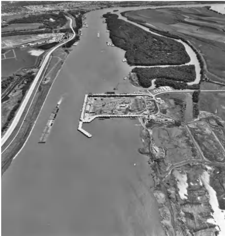
Fig. 6.13. Aerial view of the Mississippi River Lock and Dam No. 26 Replacement Project construction site near St. Louis, Missouri.
