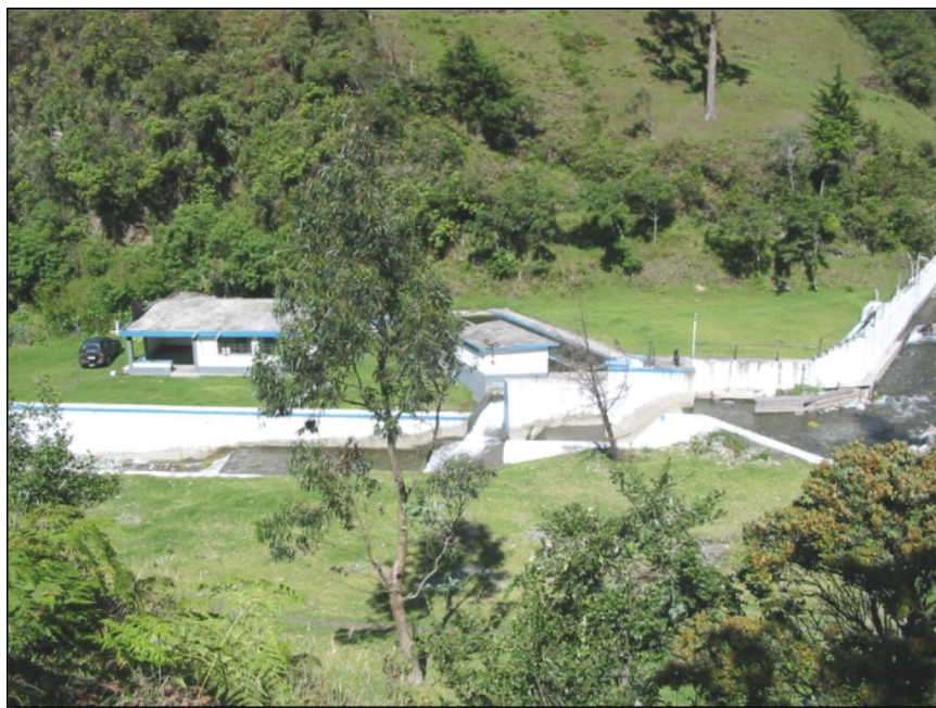
View of the existing infrastructure for the capture of water in the El Carmen creek
