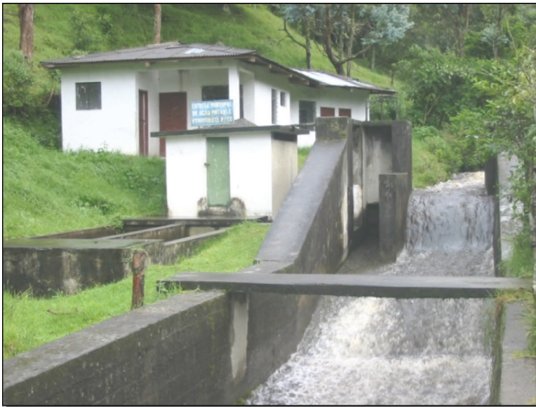
Frontal view of the San Simón catchment weir (on the left, you can see the sand catchers)
