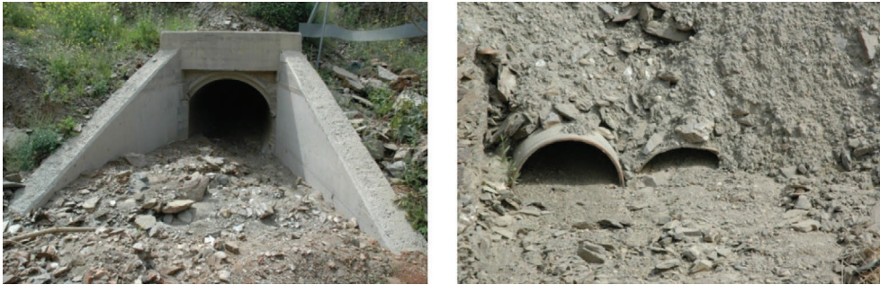
Figure 2.42 Accumulation of heterometric sediments and grounding in works of the passage of a stream
