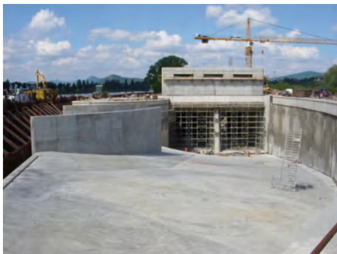
Fig. 15.7 Intake part of the SHPP Litoměřice under construction
