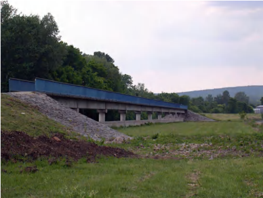
Fig. 14.11 Levee spillway at the Bulhary weir
