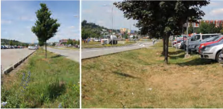
Fig. 4.5 Trench (furrow) infiltration—Campus, Brno, CR
