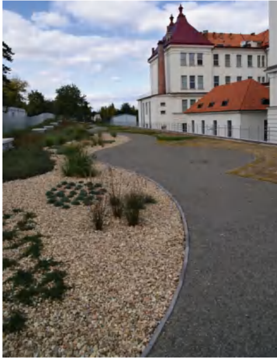
Fig. 4.1 Surface infiltration—Brno University of Technology Campus, CR
