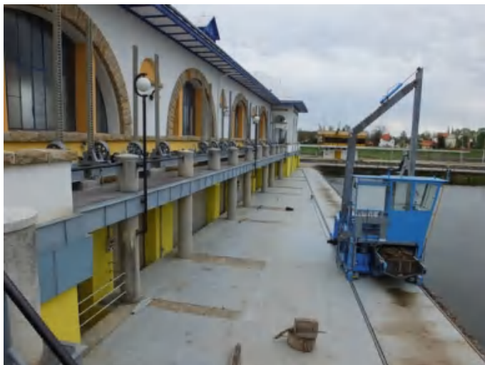
Fig. 15.14 Steel platform above the intake part of the SHPP with a new automatic cleaning machine
