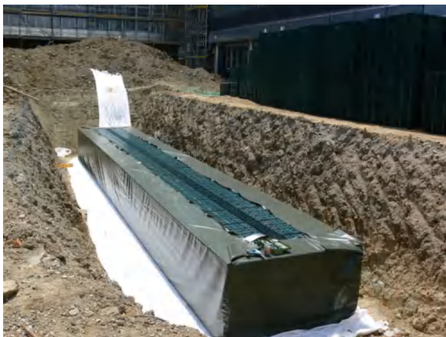
Fig. 4.12 Infiltration blocks in subsoil during construction—Campus, Brno, CR [60]
