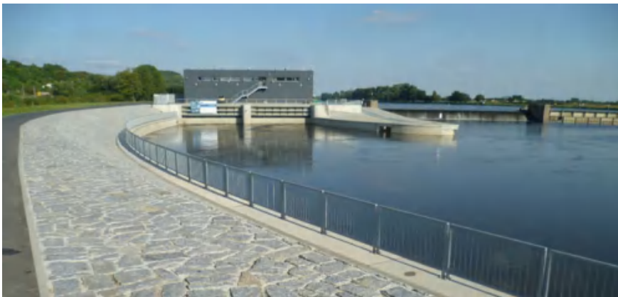
Fig. 15.4 Powerhouse of the SHPP Litoměřice from the outlet side
