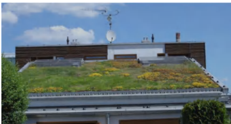
Fig. 3.3 Roof with extensive planting ( Source Kotásková )
