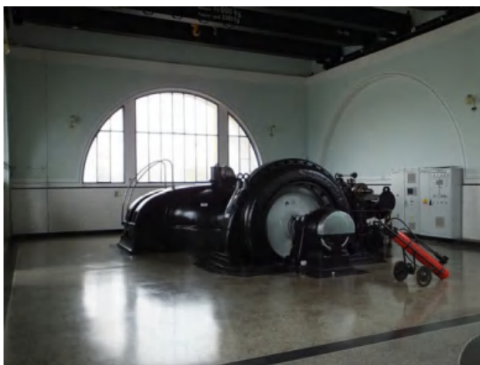
Fig. 15.15 Historical set with vertical Francis turbine in the generator hall of SHPP Mirejovice (bevel gear, generator and regulator)
