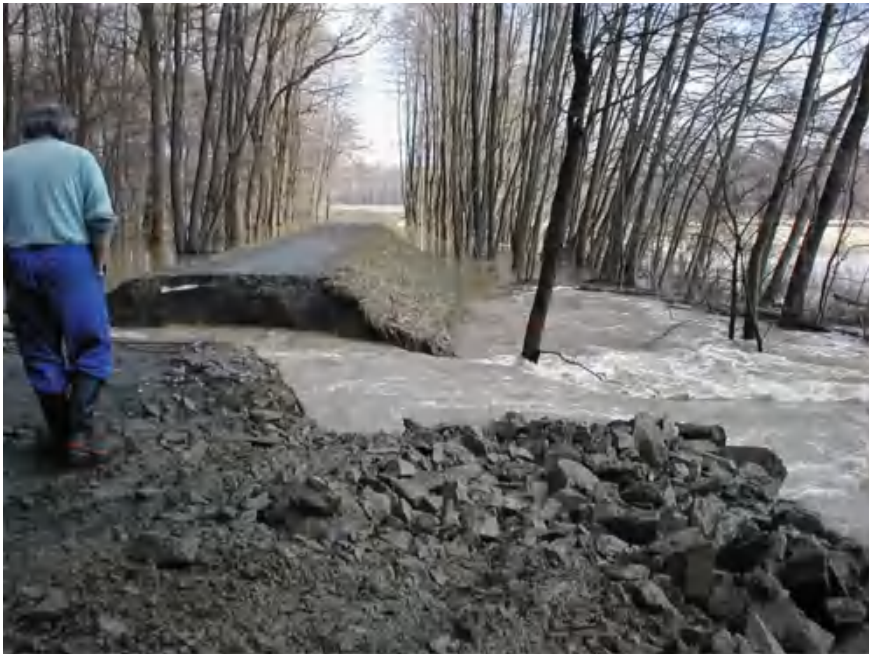
Fig. 14.3 Collapse of the Horka levee at the Morava river
