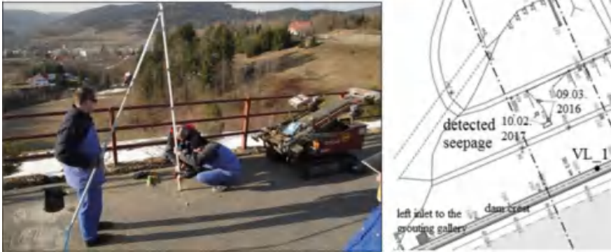
Fig. 13.7 Installation of probe VL_4 of the EIS method into the dam's sealing core (left), detected seepage sites after 2013—an outline of the situation (right)
