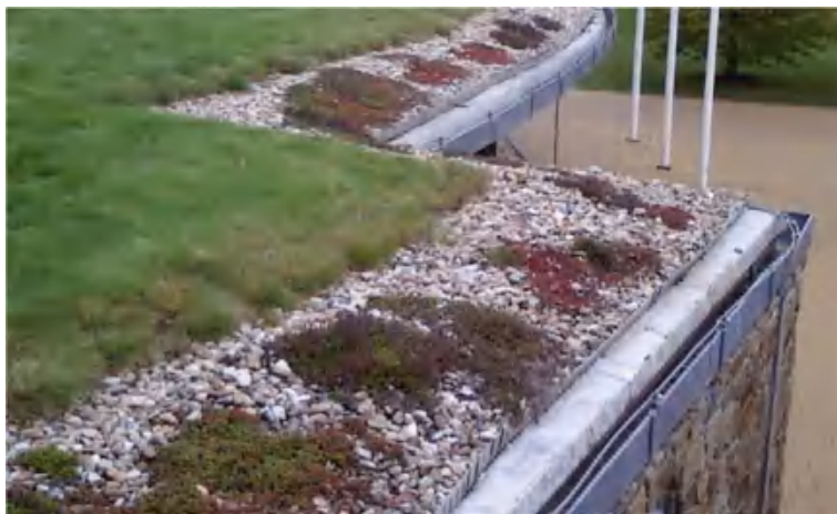
Fig. 3.5 Edge of the roof with semi-intensive planting ( Source Kotásková )
