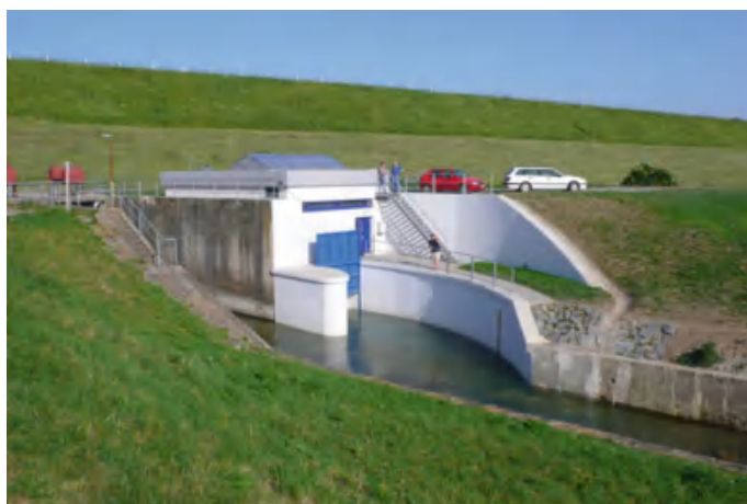
Fig. 15.19 Powerhouse of the SHPP Rozkoš from the outlet side (source Hydrohrom, s.r.o.)
