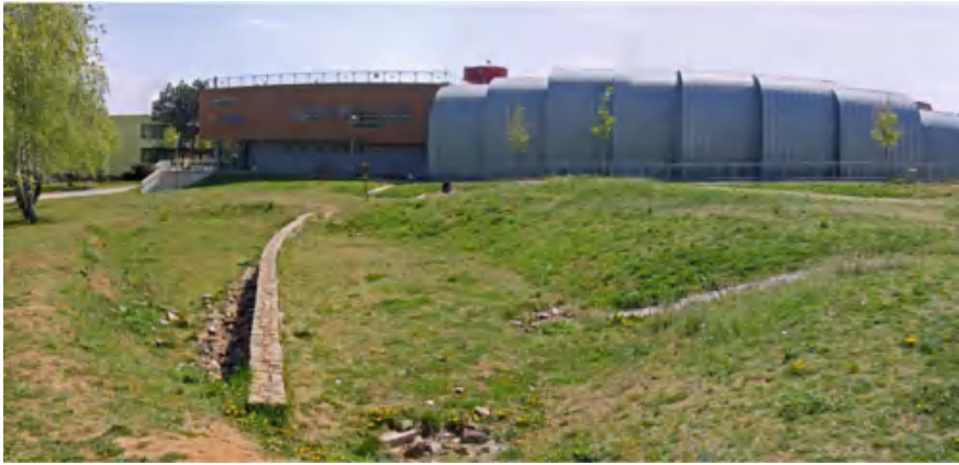
Fig. 4.3 Swale infiltration—Kohoutovice, Brno, CR
