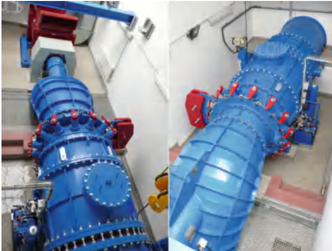
Fig. 15.23 Horizontal axial S-type Kaplan turbine in the SHPP Rozkoš (source Hydrohrom, s.r.o.)
