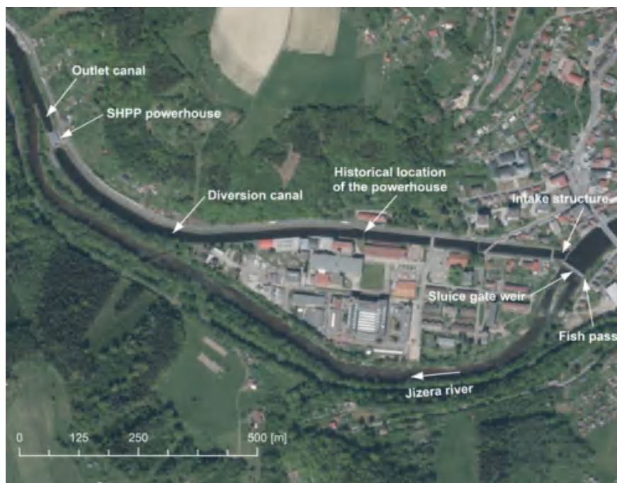
Fig. 15.29 Situation of SHPP Železný Brod (based on data [10])
