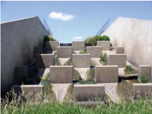
Fig. 11.16 Baffle chute energy drop structure (Wikipedia)
