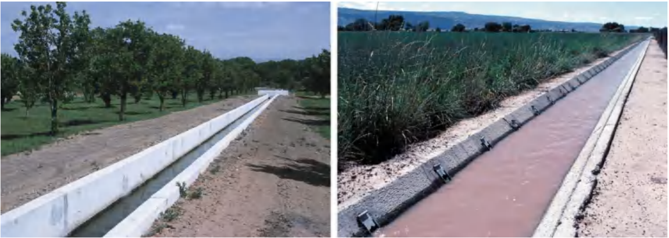
Fig. 11.1 Square and trapezoidal irrigation ditches (Credit NRCS)
