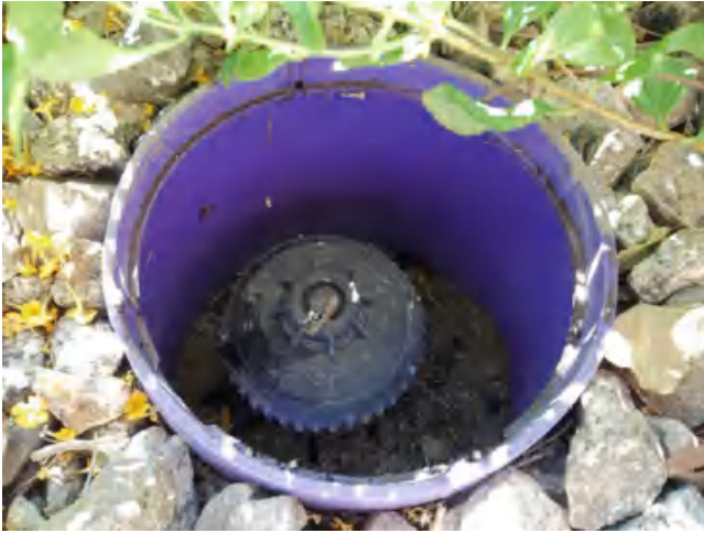
Fig. 15.4 Multioutlet emitter in valve can
