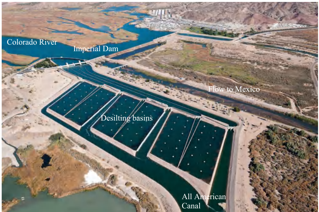
Fig. 11.2 Imperial diversion dam (Courtesy of United States Bureau of Reclamation)
