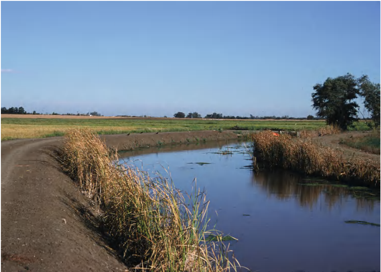
Fig. 11.7 Tailwater recovery channel (Credit NRCS Jeff Vanuga)
