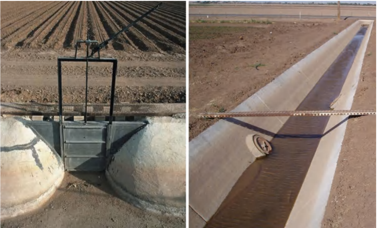
Fig. 11.5 Slide gate in farm irrigation ditch bank with energy dissipation blocks to prevent erosion ( left ) and spill ( right )
