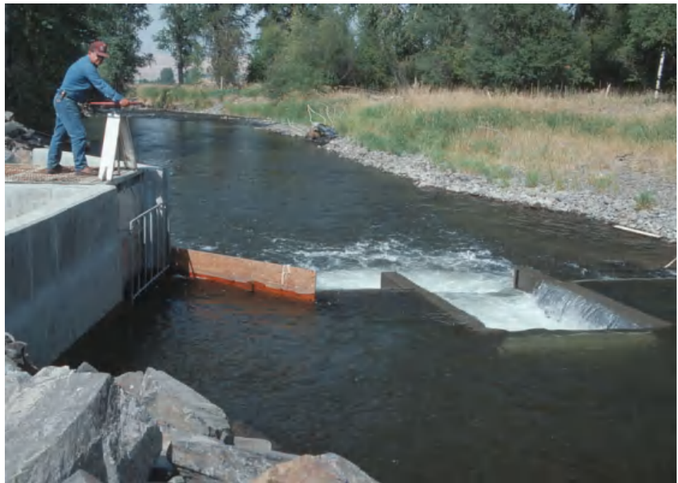
Fig. 11.4 Irrigation turnout upstream from dam in stream
