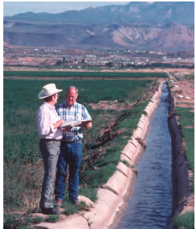
Fig. 11.8 Cracked concrete lined canal (Credit NRCS, Ron Nichols)
