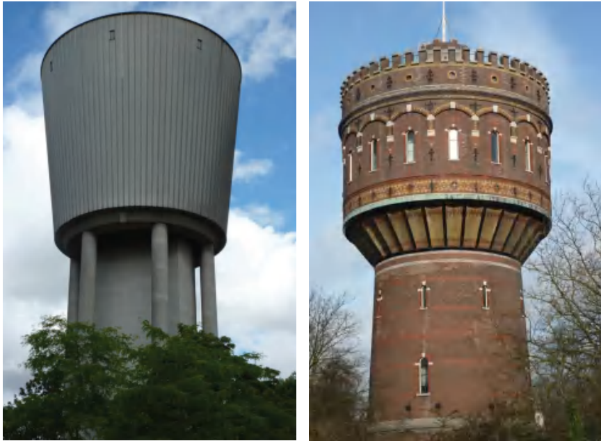
Figure 1.15 Water towers in Amsterdam (still in use) and Delft (no longer in use)
