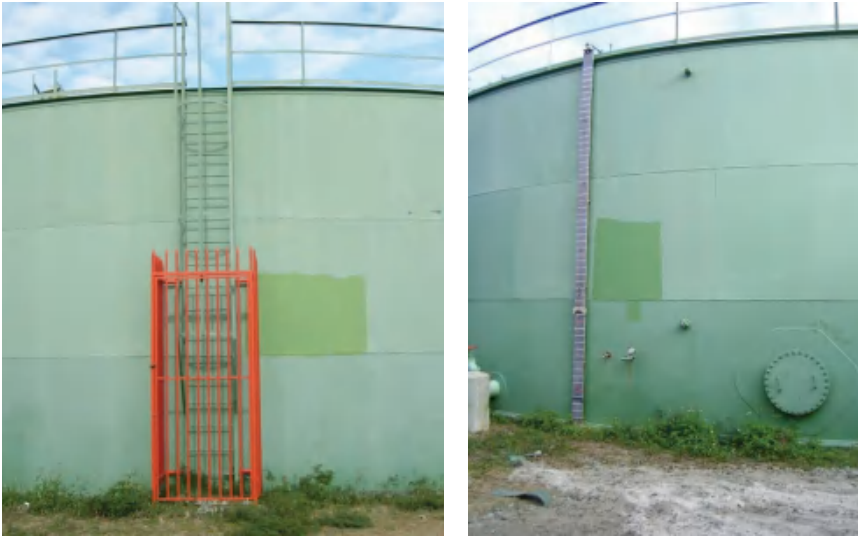
Figure 4.115 Restricted access (left-hand side) and monitoring of reservoirs water depth by float (right-hand side)
