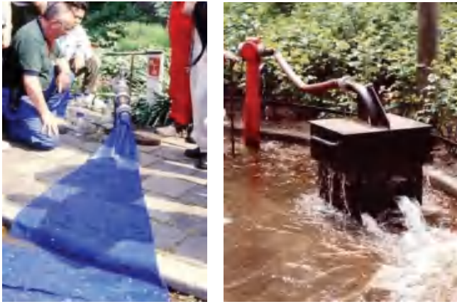
Figure 6.67 Discharge point with dampening of the water jet
