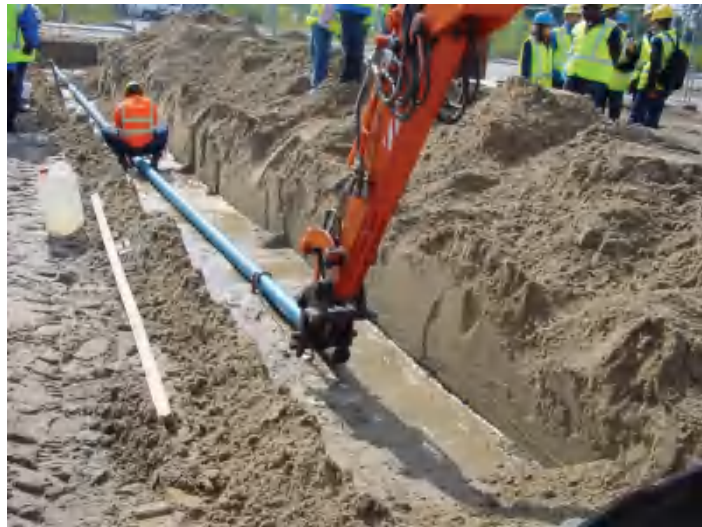
Figure 5.39 DI pipe jointing using mechanical push
