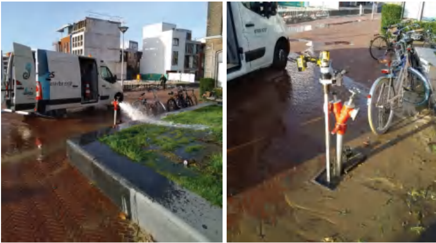
Figure 6.64. Pipe flushing process.
