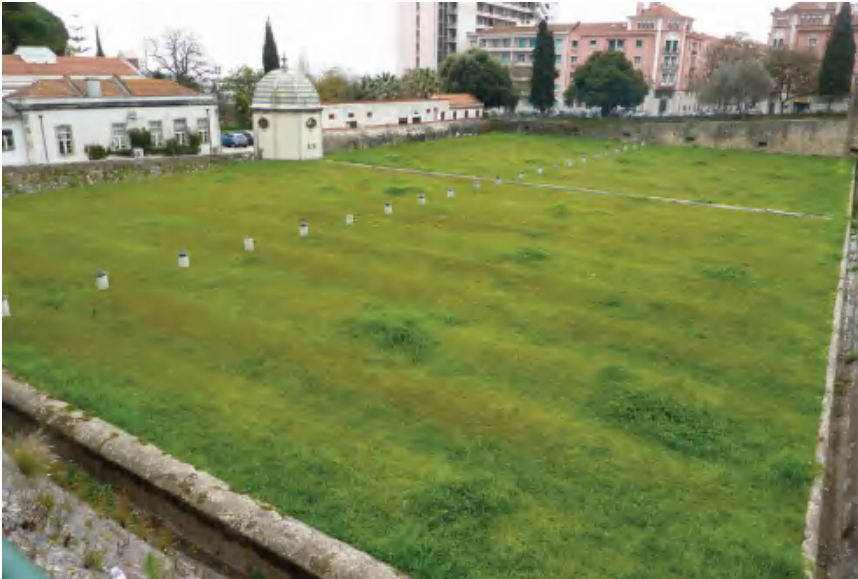
Figure 1.13 An underground reservoir in Lisbon, Portugal
