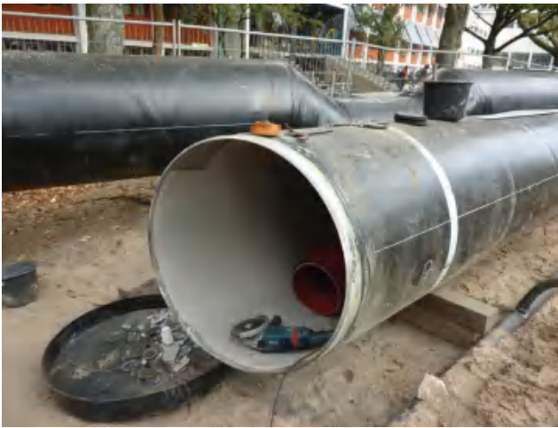
Figure 6.72 Repair of the internal cement lining of a steel pipe
