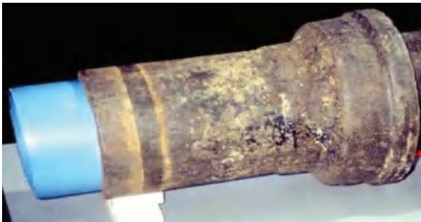
Figure 6.76 Structural relining of an old CI pipe
