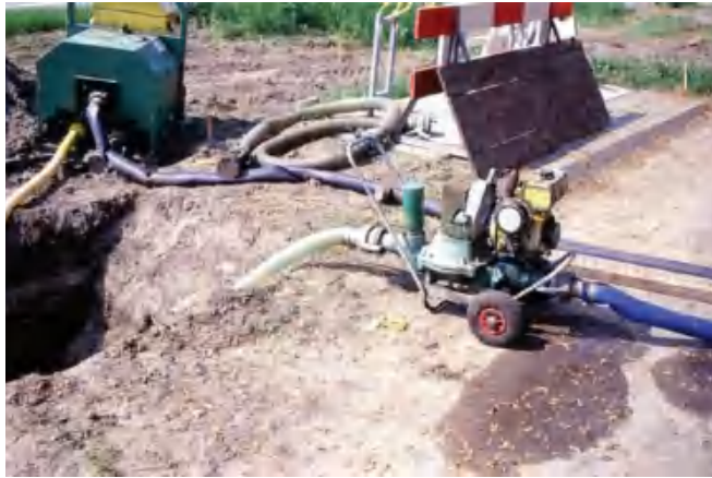
Figure 5.19 Trench dewatering by pumping
