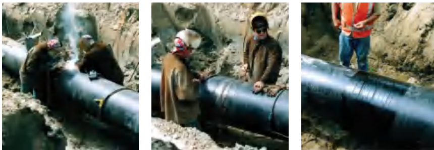
Figure 4.59 Welding of steel pipes (protection with self-adhesive tape)
