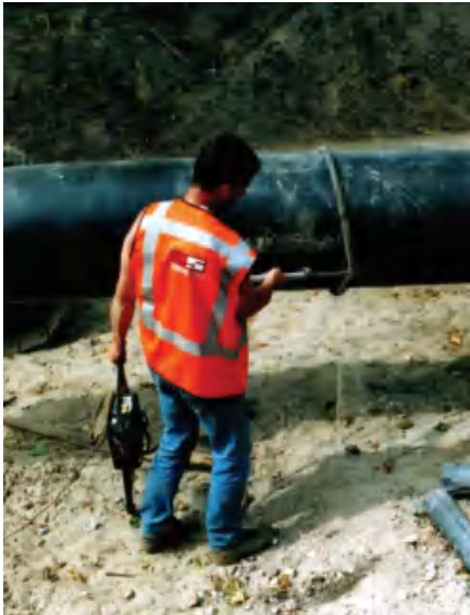
Figure 5.25 Testing of external coating
