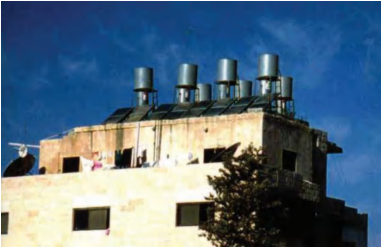
Figure 1.16 Roof tanks in Ramallah, Palestinian Authority
