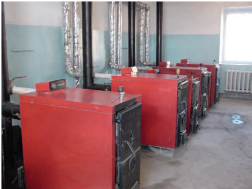
Figure 4.114 Reservoir water heating to prevent freezing during winters in Ulaanbaatar, Mongolia
