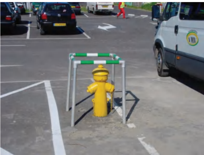
Figure 4.105 Hydrant protection against damage from parking vehicles
