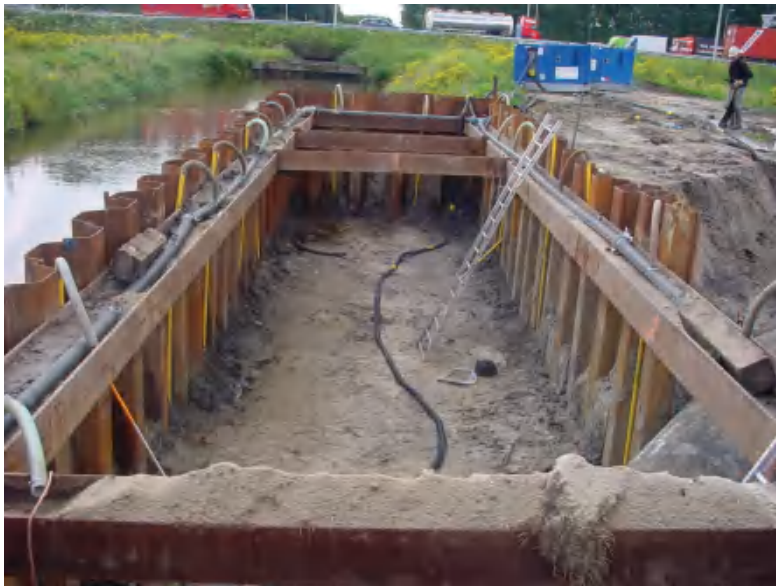
Figure 5.12 Shoring with pile-driven metal sheets
