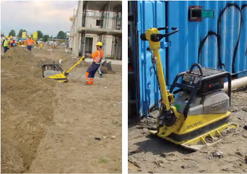
Figure 5.45. Backfilling and compacting of the trench
