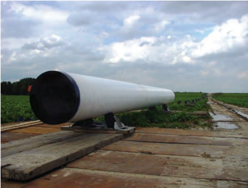
Figure 5.18 Steel pipe, D = 1000 mm, ready for laying
