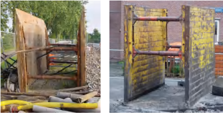
Figure 5.13 Steel boxes used for the shielding technique
