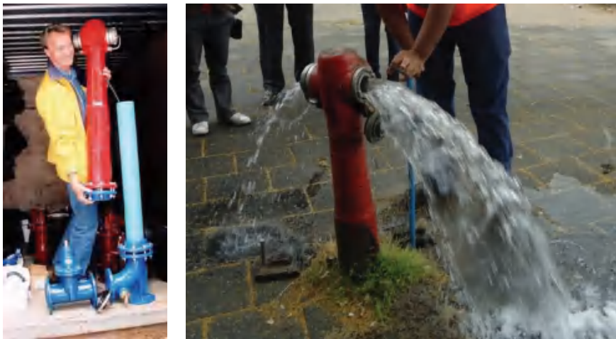
Figure 4.102. Dry barrel hydrants.
