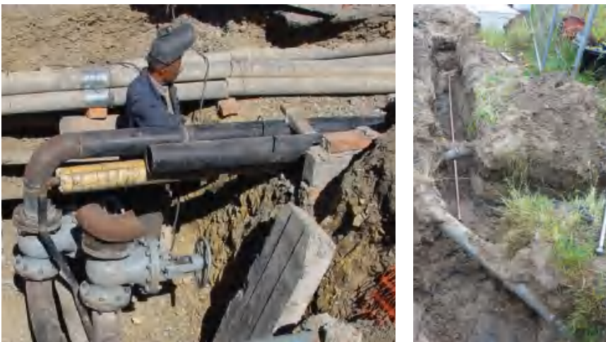
Figure 5.7 Manually excavated trenches
