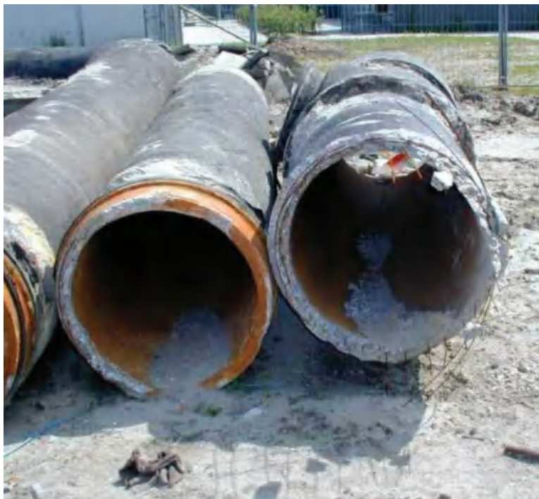
Figure 4.49 Old concrete pipes reinforced with steel net
