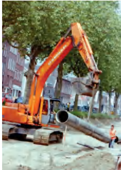
Figure 5.26 Pipe positioning in a trench
