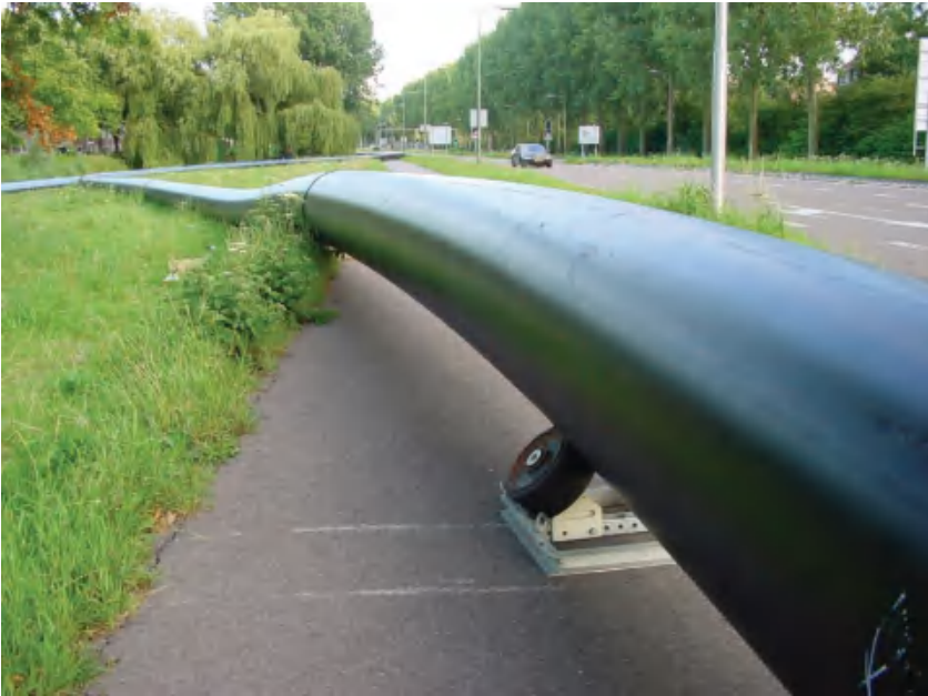
Figure 4.62 A large-diameter PE pipe section with joints created by the butt-fusion method
