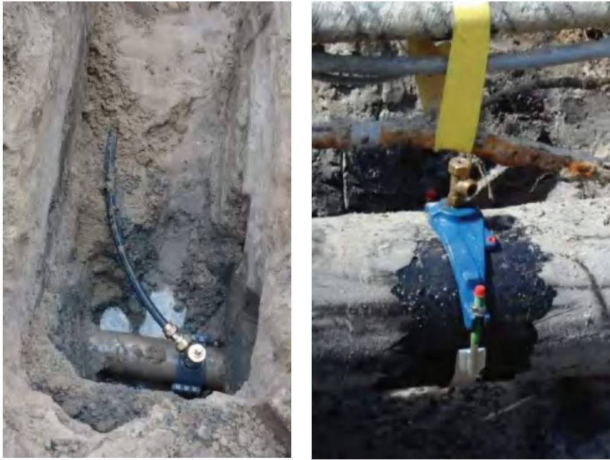
Figure 4.109 PVC (left) and DI pipe (right) saddles commonly used for vertical service connections in the Netherlands
