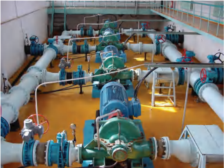
Figure 1.20 Horizontal centrifugal pumps
