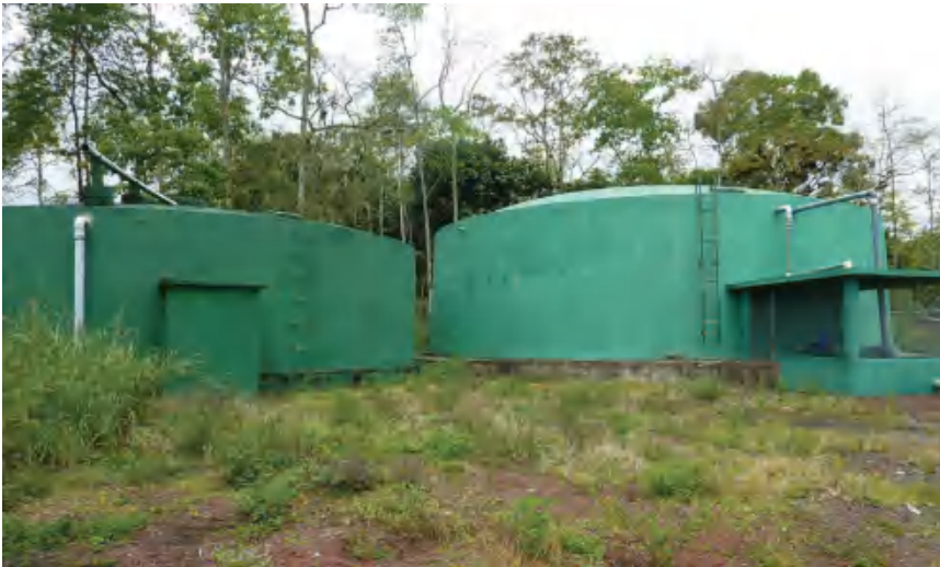
Figure 1.14 Ground level concrete reservoirs in Galápagos, Ecuador
