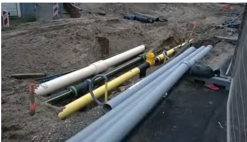
Figure 5.2 Simultaneous laying of drinking water, sewage, and gas pipelines
