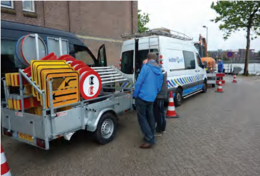
Figure 5.3 Signs for traffic regulation during network construction Courtesy: Waternet, Amsterdam.
