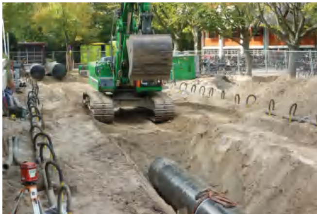
Figure 5.21 Application of the wellpoint method
