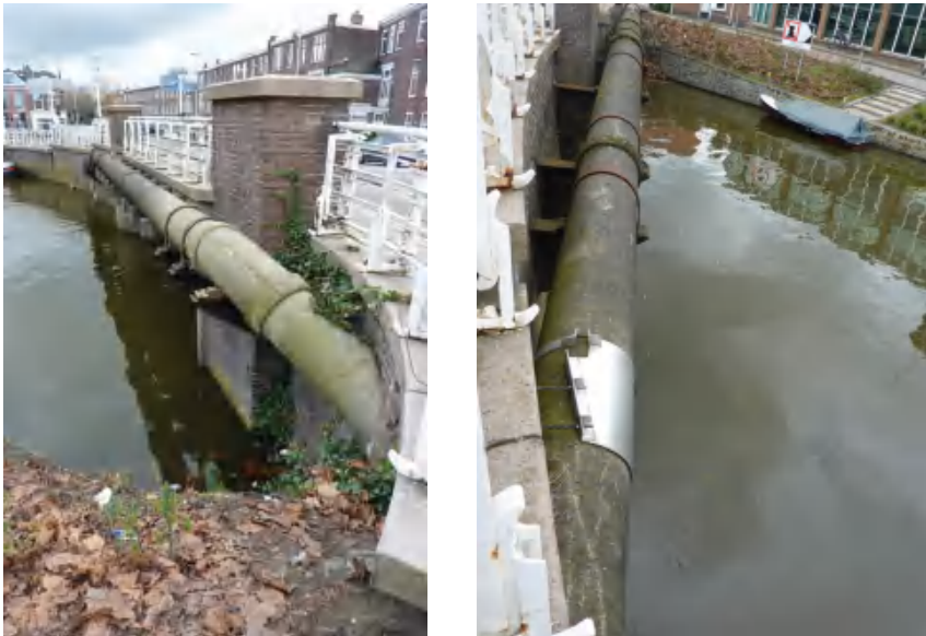
Figure 5.35 Concrete pipe laying at a bridge
