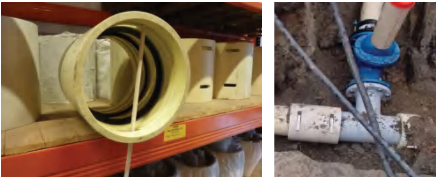
Figure 4.68 Dual socket joint for PVC pipes, with additional strengthening
