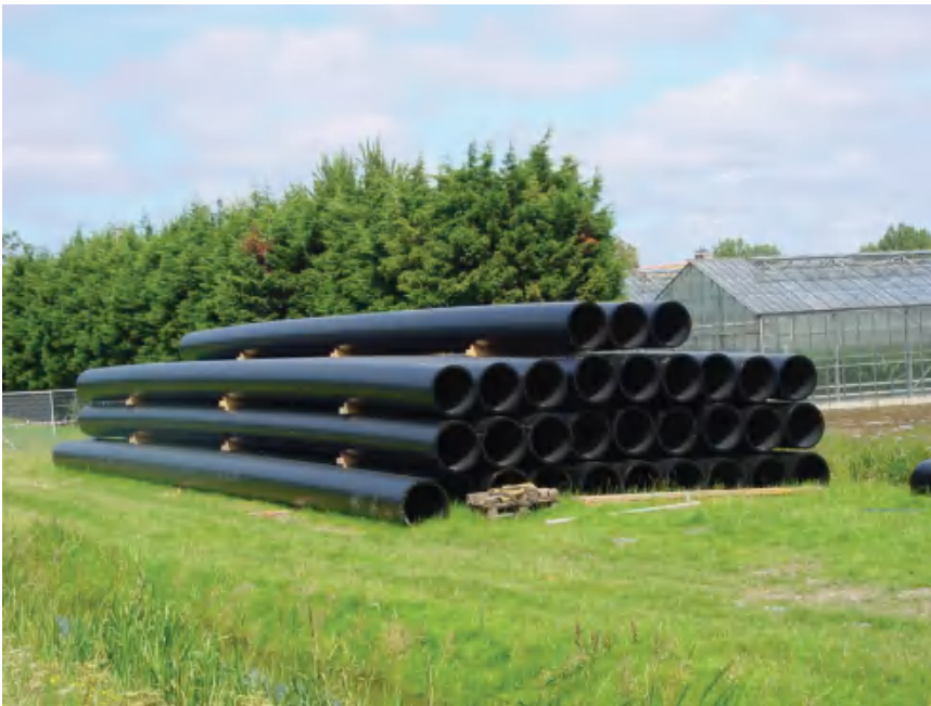
Figure 5.4 Proper stacking of PE pipes
