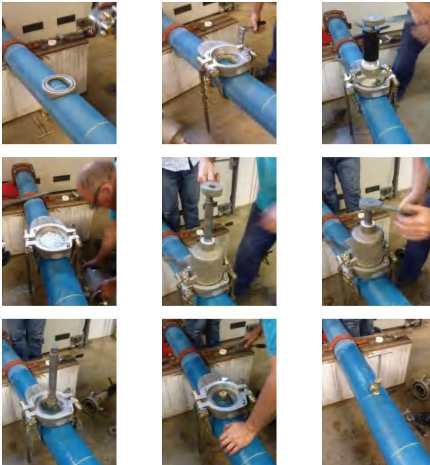
Figure 4.108 Service connection without a saddle on DI pipes
