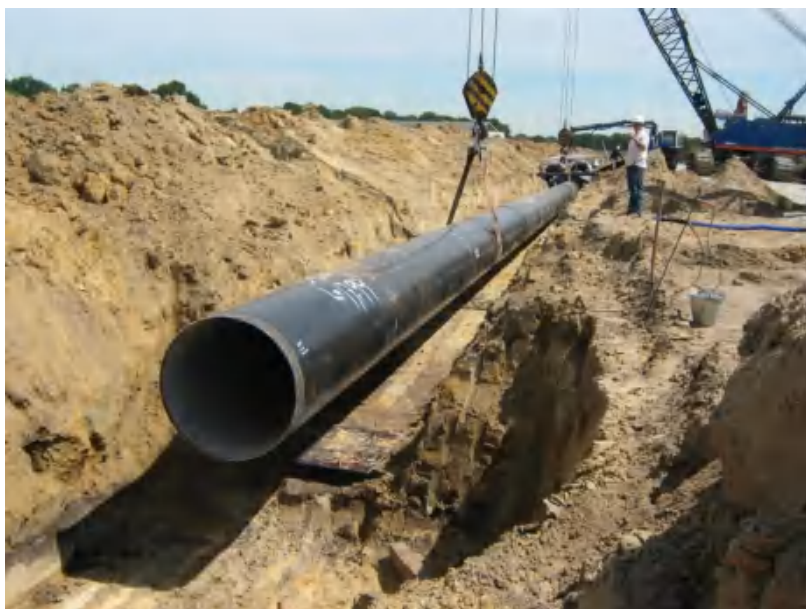
Figure 4.42 A cement-lined steel pipe with PE coating
