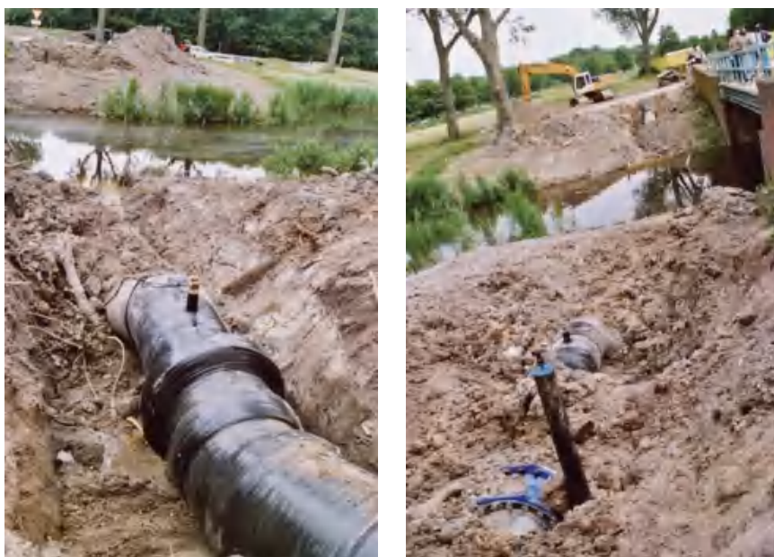
Figure 6.59 Cathodic protection applied to steel pipes
