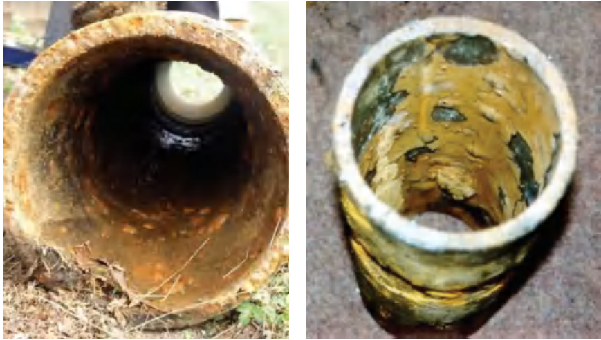
Figure 4.35 Old cast iron pipes in reasonably good condition
