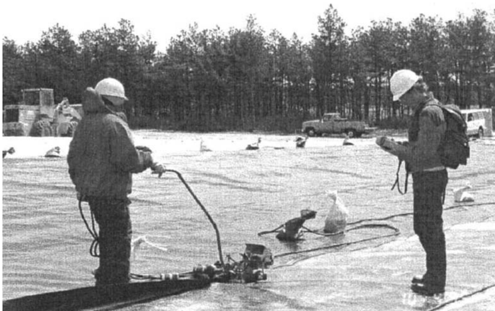
FIGURE 37.9 Monitoring seaming of a geomembrane liner.
