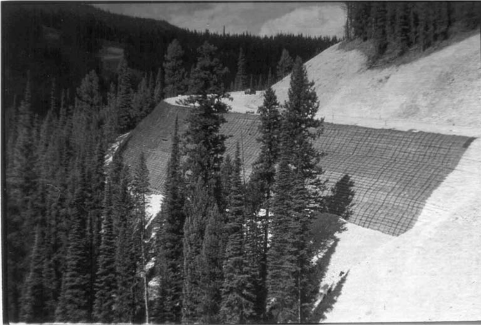
FIGURE 37.16 Erosion control mat placed to help establish the vegetation on the face of a 1H:1V reinforced soil slope.
