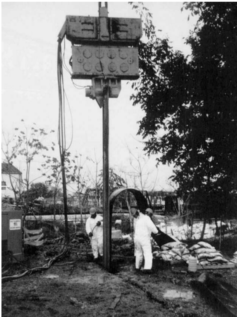
FIGURE 37.20 Installation of HDPE barrier wall utilizing conventional pile driving equipment. (Photo courtesy of Groundwater Control Inc.)
