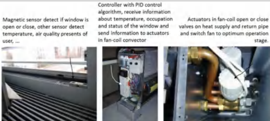
Fig. 8.36 Sensors and actuators for control of fan-coil
