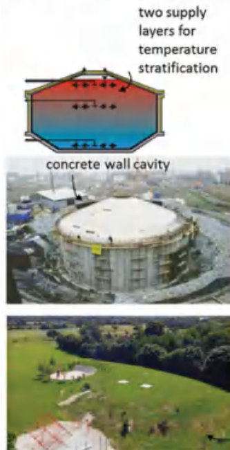
Fig. 8.11 Examples of long-term water (left) and pit-type seasonal heat storage (right) (SDHplus 2015)
