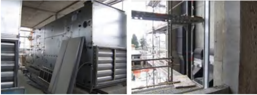
Fig. 8.23 AHU on the roof of the office building (left); vertical channels for supply of ventilation air (right)
