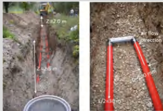
Fig. 11.36 U-shaped ground heat exchanger
