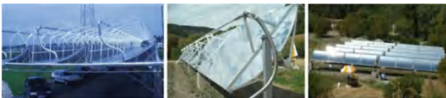
Fig. 9.10 Parabolic CSC with area 32 m 2 that drives double stage absorption chiller with rated cooling power of 16 kW (left), (Broad Technology Centre, China) 180 m 2 CSC array of the double-stage chiller with cooling power of 116 kW [middle, right; Lokurly 2010]
