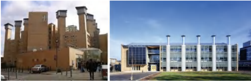
Fig. 11.3 Examples of natural ventilated buildings with stack enhance natural ventilation; Library and Resource Centre Coventry University (left) (Limam et al. 2011), BRE Office building (right) (Kleiven 2004)
