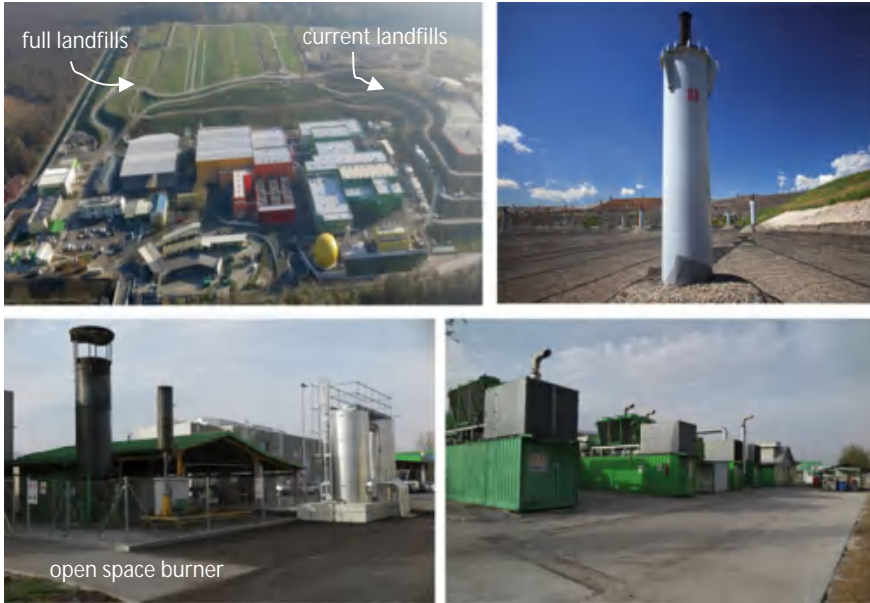
Fig. 2.22 Centre for solid waste treatment of Municipality of Ljubljana that will replace landfills in the future (top, left); landfill ready for municipal solid waste disposal with water-tight membrane and set of degassing shafts (top, right); landfill gas pumping station with open burners where landfill gas is burned if the content of methane in the landfill gas is lower than 40% or during the maintenance (bottom, left); system of landfill gas power plants as cogeneration units; unit can produce electricity and heat if the amount of methane in landfill gas is above half of designed value (bottom, right) (Trivunčević 2016)
