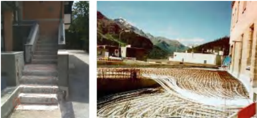
Fig. 8.32 Stairs heated with electrical resistant heater (left); ground heating of pavement in St. Moritz; in this case, heating water must be mixed with antifreeze fluid (right)
