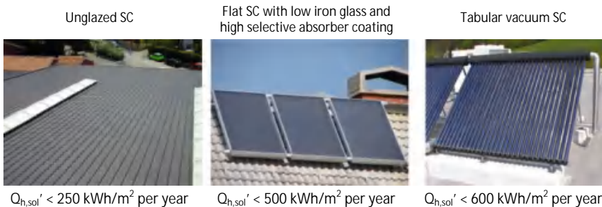
Fig. 6.29 Specific generated heat Q_{h, sol'} of different types of STC; values are established for the optimum positions of STC
