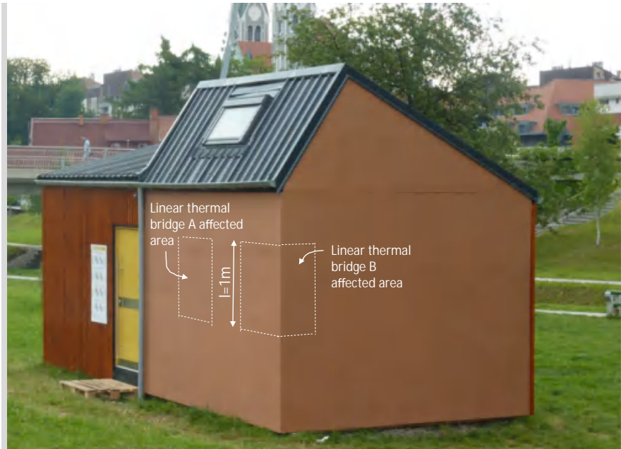
Fig. 3.11 Photo of Virtual Lab building with impact area of analysed thermal bridges
