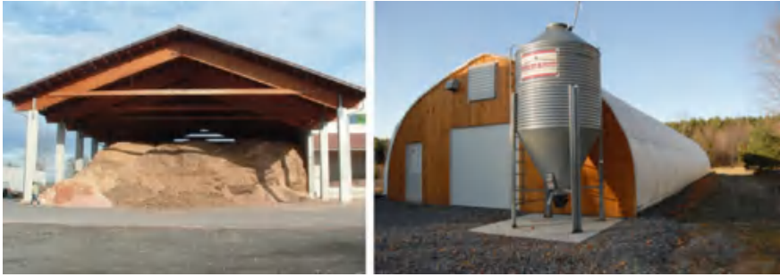
Fig. 2.21 Outdoor storage for wood chips (left); outdoor silos for pellets (right) ( www.mywoodpelletsolution.com )
