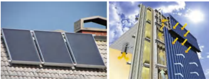
Fig. 6.23 Liquid flat plate solar thermal collectors (left) in close loop solar heating system; air solar thermal collector in form of perforated facade cover layer for preheating ventilation supply air (right ( solarwall.com ))
