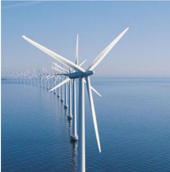
Fig. 2.4 Low energy density is one of the drawbacks of RES; one turbine presented on the picture with rotor diameter of 70 m, has power of electricity generator comparable with mechanical power of the motor of F1 racing car; despite that, electricity production by wind turbines is cost effective especially with off shore applications because of the higher wind speeds in comparison to those on the land ( http://wonderfulengineering.com/38-high-def-wind-turbine-pictures-from-around-the-world/ )
