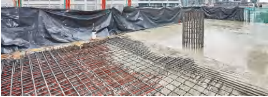
Fig. 8.31 Pipes built-in in the core of the concrete-bearing plate in office building; circulation pipes must be installed in TABS during the construction of the building ( www.rehau.com )
