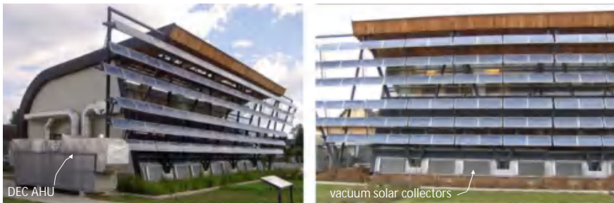
Fig. 9.31 DEC solar cooling system for space cooling of office building; AHU has rated capacity of 6000 m 3 /h and rated DEC cooling power is 30 kWc; heat for dehumidification of the desiccant wheel is delivered by vacuum solar collectors array with area of 12 m 2 ; DEC system produce 10,000 kWh of cold at seasonal coefficient of performance 0.6 . ( www.oekoplan-hartberg.at )
