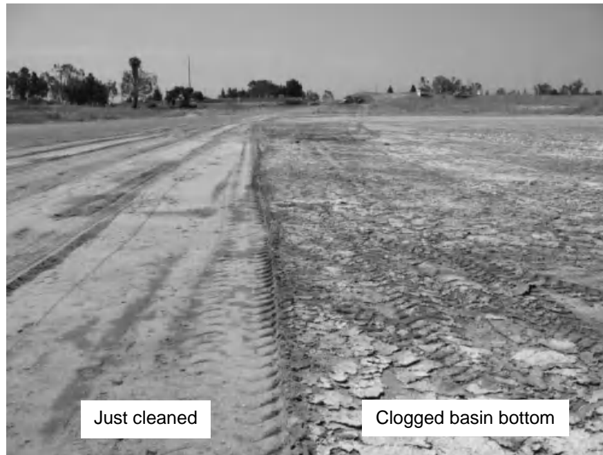
FIGURE 6-3 Clogging layer in recharge basin operated in Orange County, California, adjacent to cleaned portion of recharge basin where the clogging layer was removed. Photo courtesy of Adam Hutchinson, Orange County Water District.
