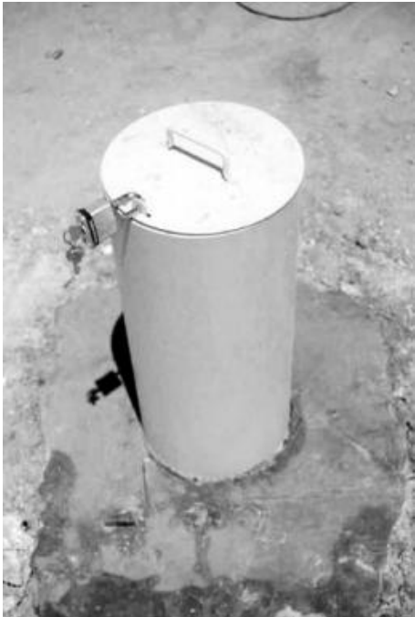
FIGURE 10.134 A case-hardened steel lock on the lid of the protective casing provides adequate security under most conditions.
