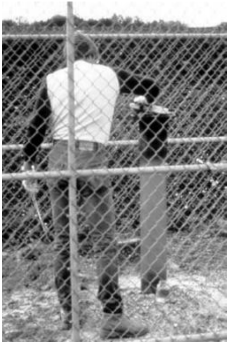
FIGURE 10.135 In areas where a high level of security is required, it may be necessary to provide a locked, fenced-in enclosure for the well.
