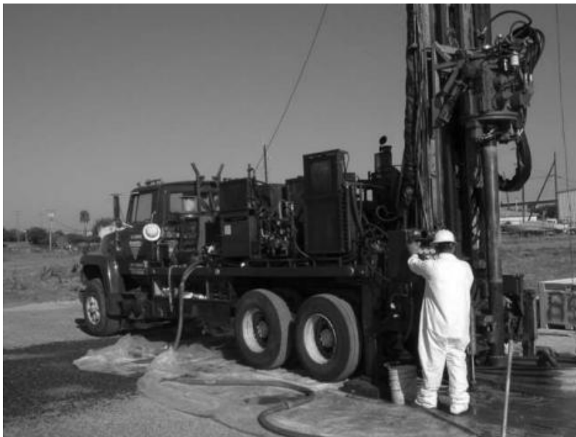
FIGURE 5.8 Sonic drilling rig.
