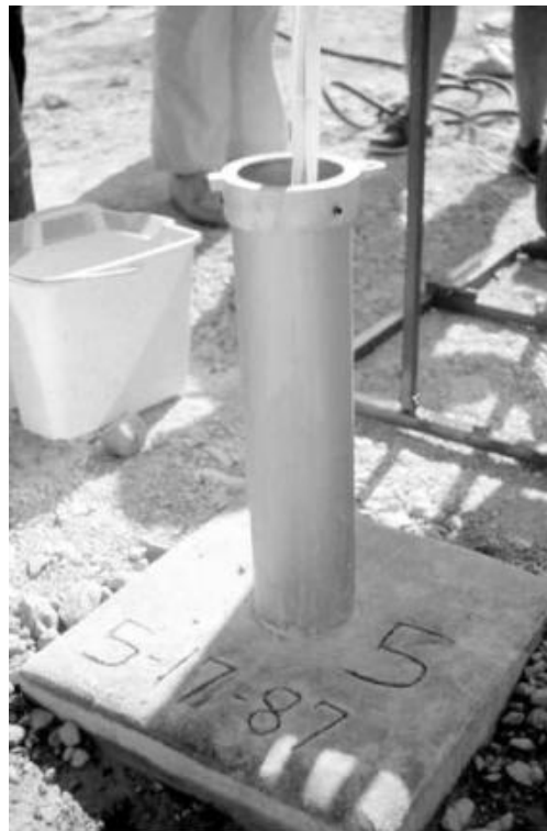
FIGURE 10.152 Occasionally, the monitoring well identification may be marked into the concrete surface seal.
