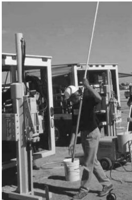
FIGURE 10.33 Installation of a prepacked well screen using a direct-push machine.
