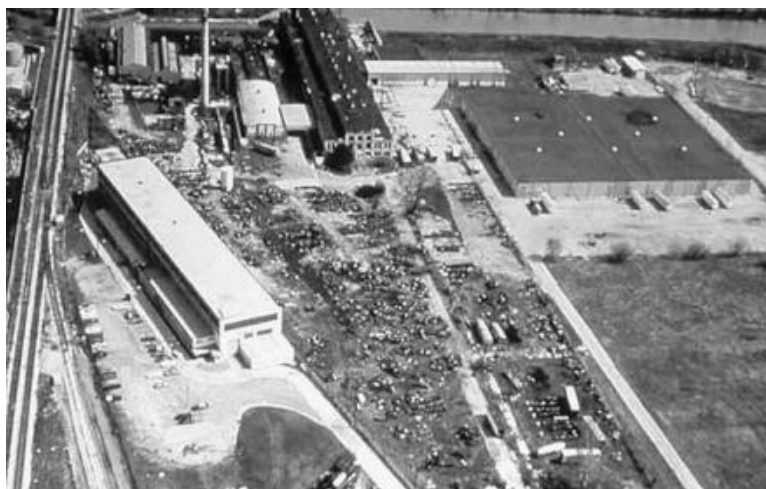
FIGURE 2.4 Most uncontrolled hazardous waste sites that once stored thousands of drums of toxic materials have been identified and the worst have been placed on U.S. EPA's National Priority list, a program initiated under CERCLA (better known as Superfund). However, at least a few dozen new sites are discovered every year, requiring site characterization in preparation for cleanup.
