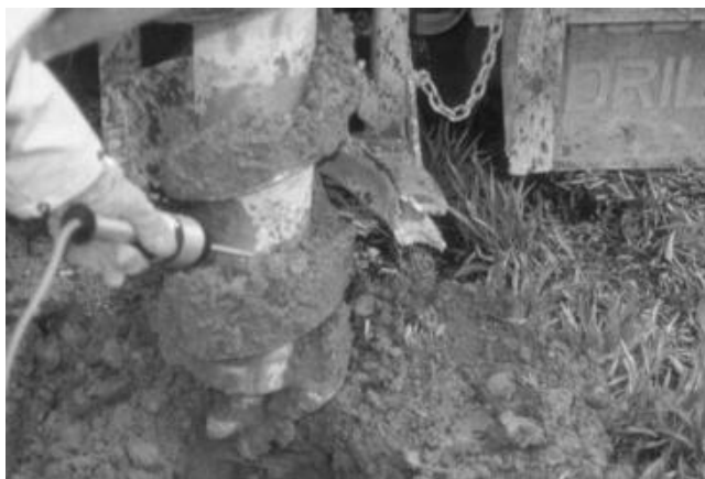
FIGURE 19.4 Air monitoring is an essential component of an HASP.
