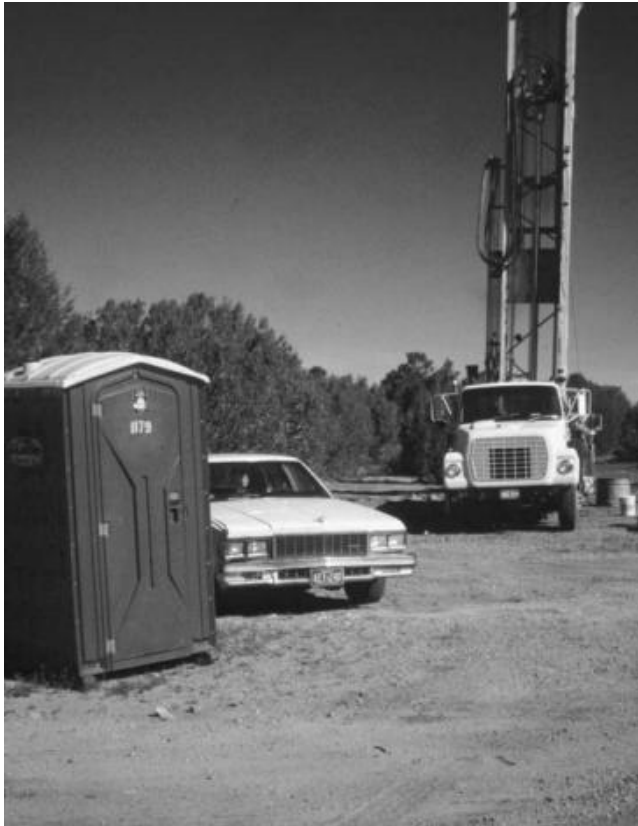
FIGURE 19.1 Field sanitation is an OSHA requirement.
