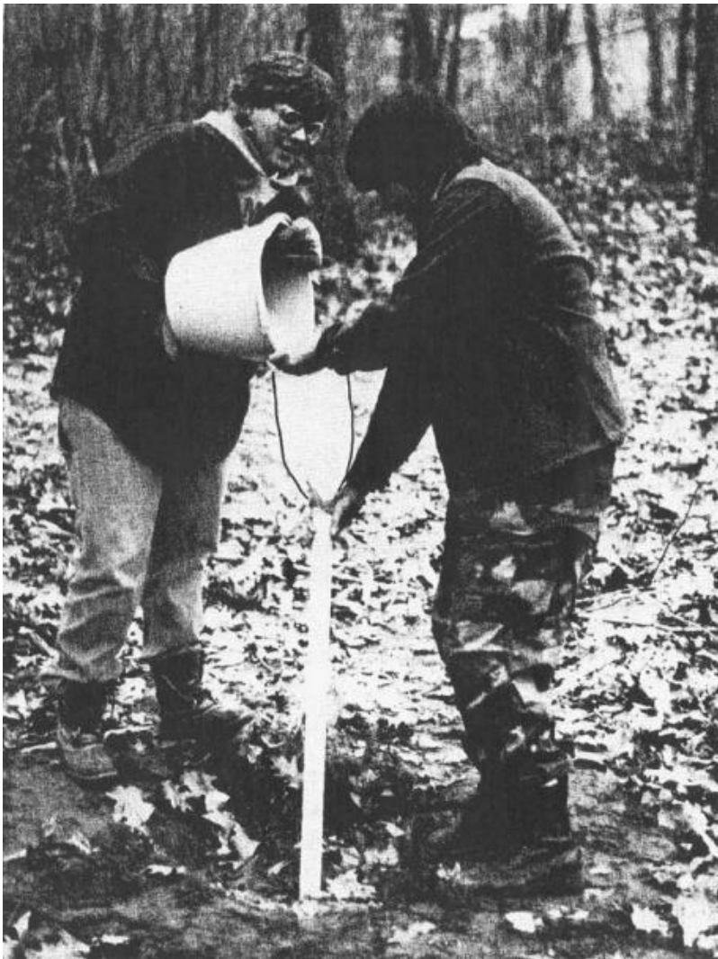
FIGURE 12.5 Filling a 2-in. monitoring well with granular bentonite.
