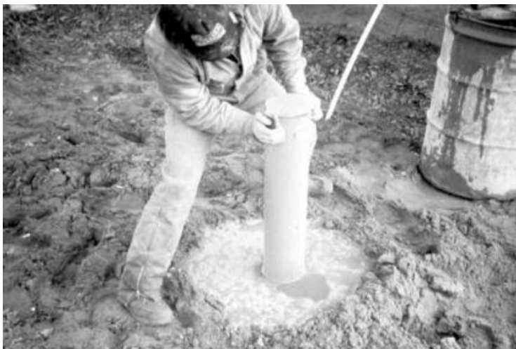
FIGURE 10.129 Installing a protective casing in the concrete surface seal.
