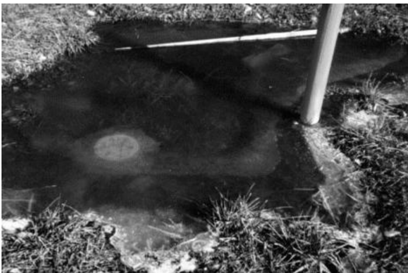
FIGURE 10.146 Flush-to-grade completions should not be used in areas where ponding or flooding occur.
