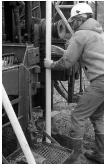
FIGURE 10.47 Installation of well casing and screen materials in a drilled borehole.
