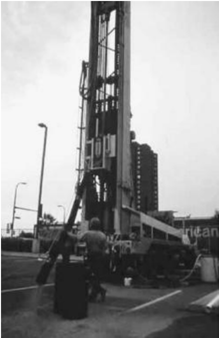
FIGURE 10.37 Air rotary with a casing hammer can be used to install monitoring wells in both unconsolidated materials and bedrock.
