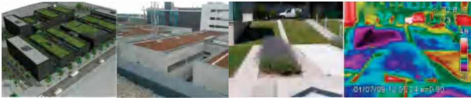
Figure 4. Sustainable drainage urban systems (SDUS) to reduce the urban heat island (UHI). Model and development of green roof on the Parc Bit building, Palma de Mallorca, Spain. Example of thermography to track the UHI evolution.
