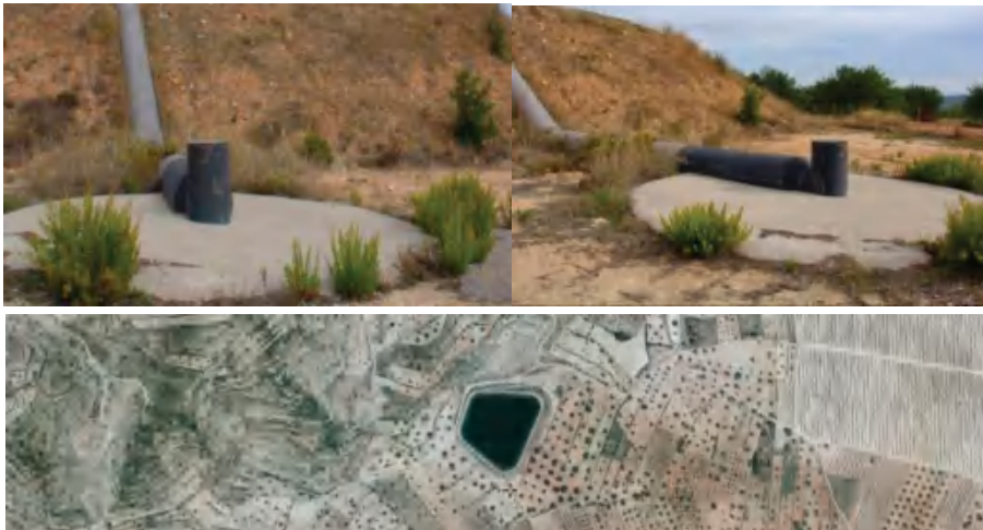
Figure 9. Deep borehole “Arnachos” at Balsa del Campo, Valencia (UTM 685,744/4,391,256) located in the margin of an irrigation pond and used as both, a safety and recharge element. Photos courtesy of J.M. Montes and FEGA.
