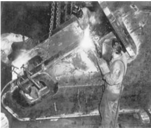
FIGURE 1.2 Long delivery time prompted welding of this cast iron punch-press frame.
