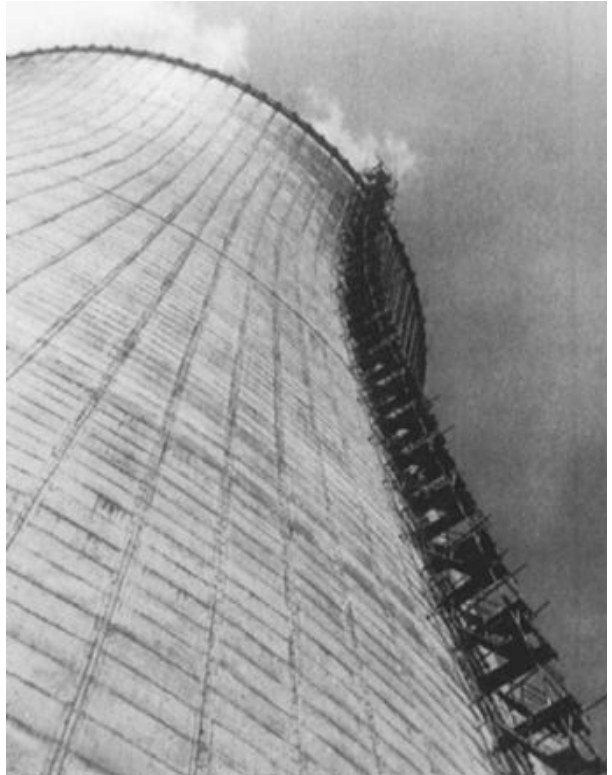
FIGURE 5.6 “Tubelox” tube and coupler scaffolding with integral step units for access to 330-ft-high curved stack. The step units are available with guardrail and midrail panels, plus the opportunity of positioning landing or rest platforms at any desired level.
