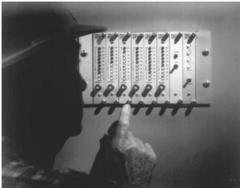
FIGURE 3.1 Valve-flow monitoring system.
