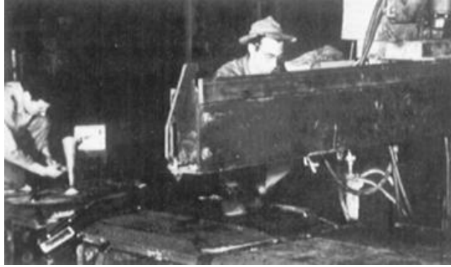
FIGURE 1.41 Steel-mill coke pushers being hard-faced by submerged arc process. Mild-steel wire and alloy flux. Fully automatic equipment in foreground, semiautomatic in background.
