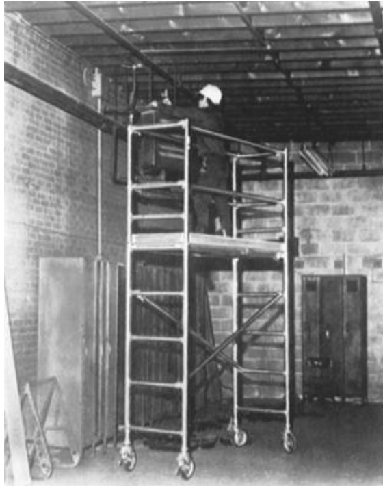
FIGURE 5.10 Aluminum ladder scaffold. Basic unit consists of 6-ft ladder frames, diagonal braces, platform, and adjustable casters. Note use of guardrails, midrails, and toeboards.
