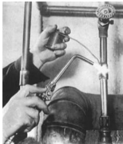
FIGURE 2.7 Soldering 1-in. copper tubing and fitting with precast holes.
