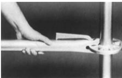
FIGURE 5.11 Preliminary step in connecting a QES™ horizontal to a prespaced ring module of a post. The horizontal's slots are merely aligned with any one of the ring slots. (Photo by Bill Mitchell.)
