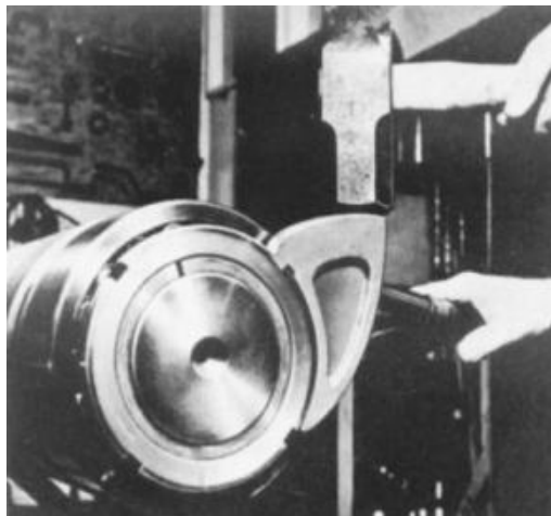
FIGURE 2.29 Use of impact-type spanner wrench.
