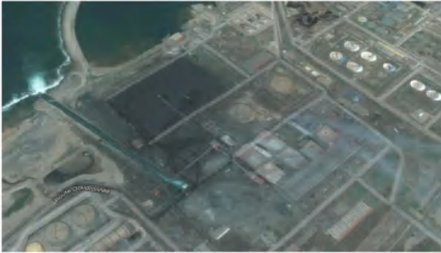
Fig. 9. A satellite image of Mohammedia Thermal Power Station.
