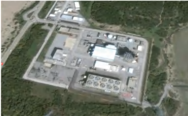
Fig. 8. A satellite image of Tahaddart Thermal Power Station.
