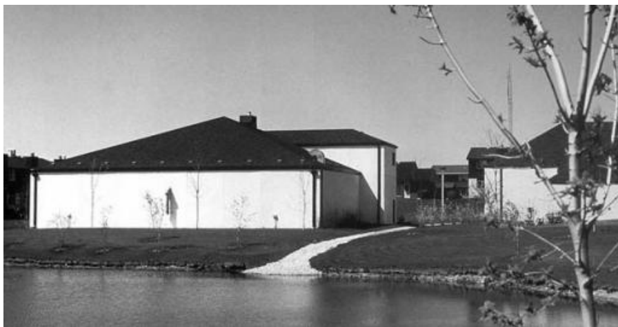
Fig. 27-5. Disguised concrete tanks
