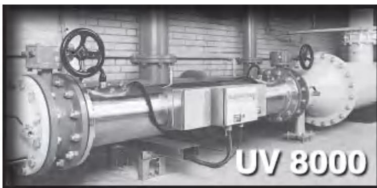
Fig. 19–16. Closed vessel UV reactor (Courtesy of Trojan Technologies Inc.)
