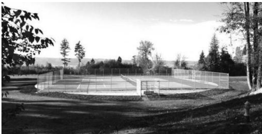
Fig. 27-3. Combined use tank site (Courtesy of DYK, Inc.)
