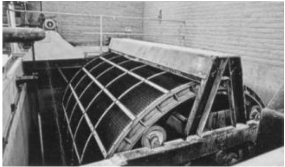
Fig. 8-12. Microscreen installation (Courtesy of USFilter-Rex and LinkBelt Intake Products)
