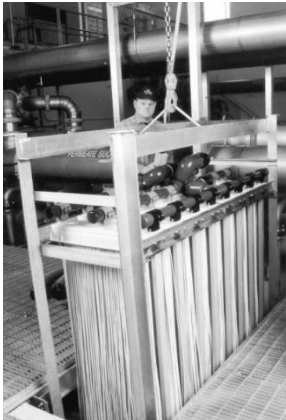
The modular filter rack is easily removed from the filter cell for convenient maintenance.
