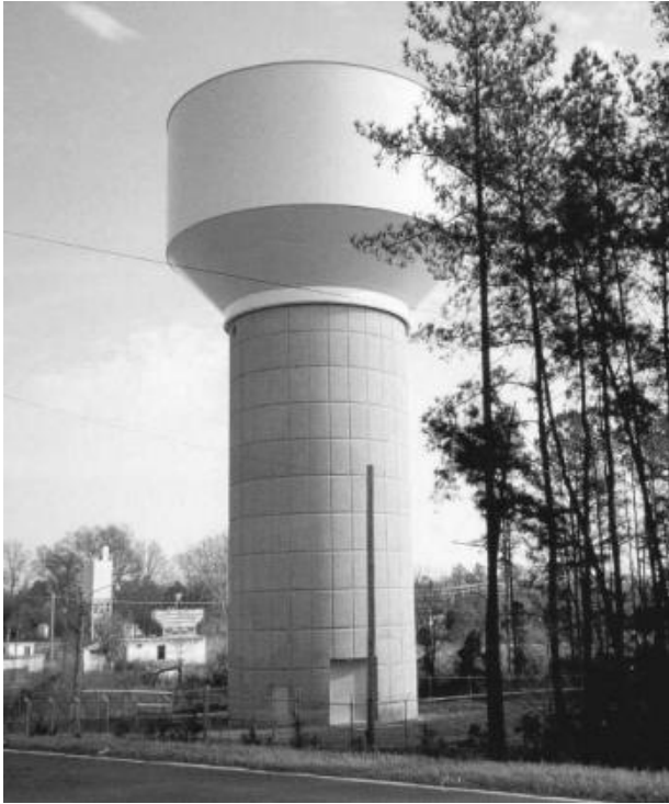
Fig. 27-6. Elevated concrete and steel tank
