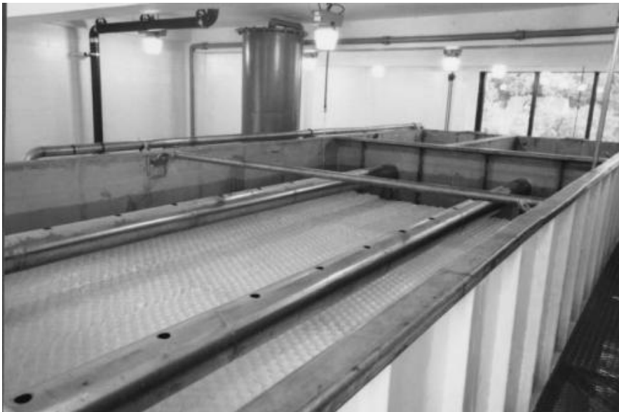
Fig. 25-18. Photo of Pulsapak package water treatment plant. (Courtesy of Infilco Degremont, Inc.)
