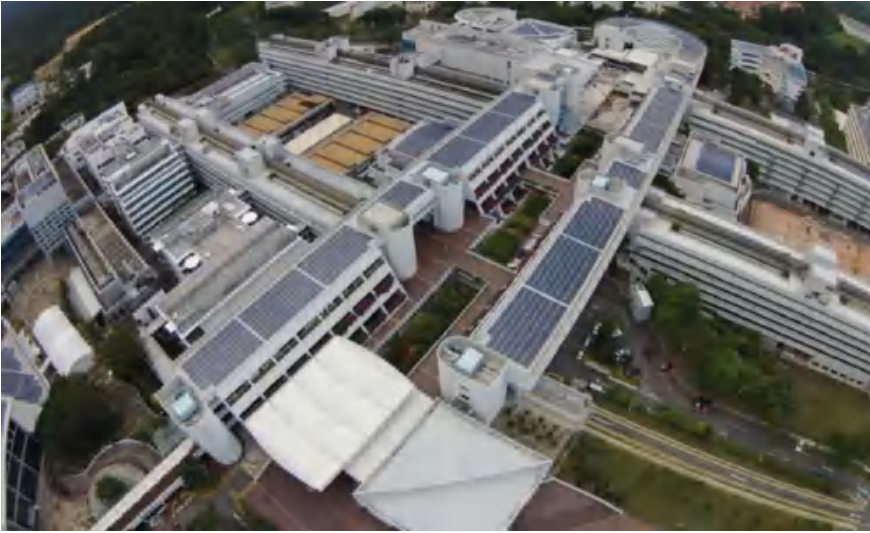
Fig. 7.1 Photo of solar panels installed on the rooftop of the NTU campus buildings in Singapore
