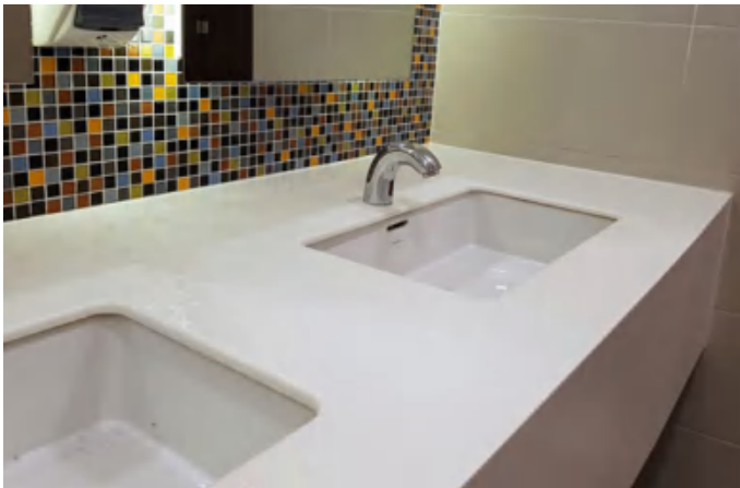
Fig. 8.2 Photo showing a sensor controlled water tap
