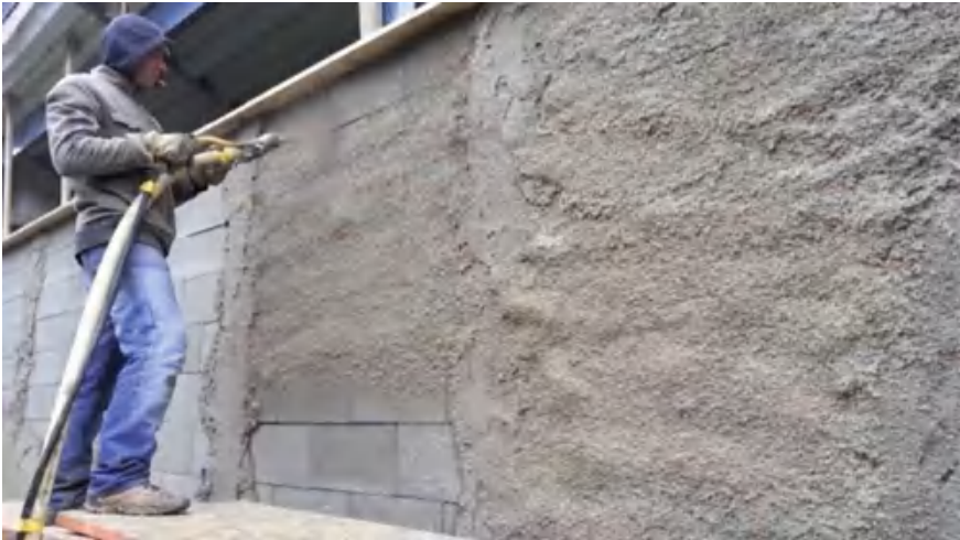
Fig. 4.9 Photo showing application of a thermal insulation plaster (MagorTherm 2015)
