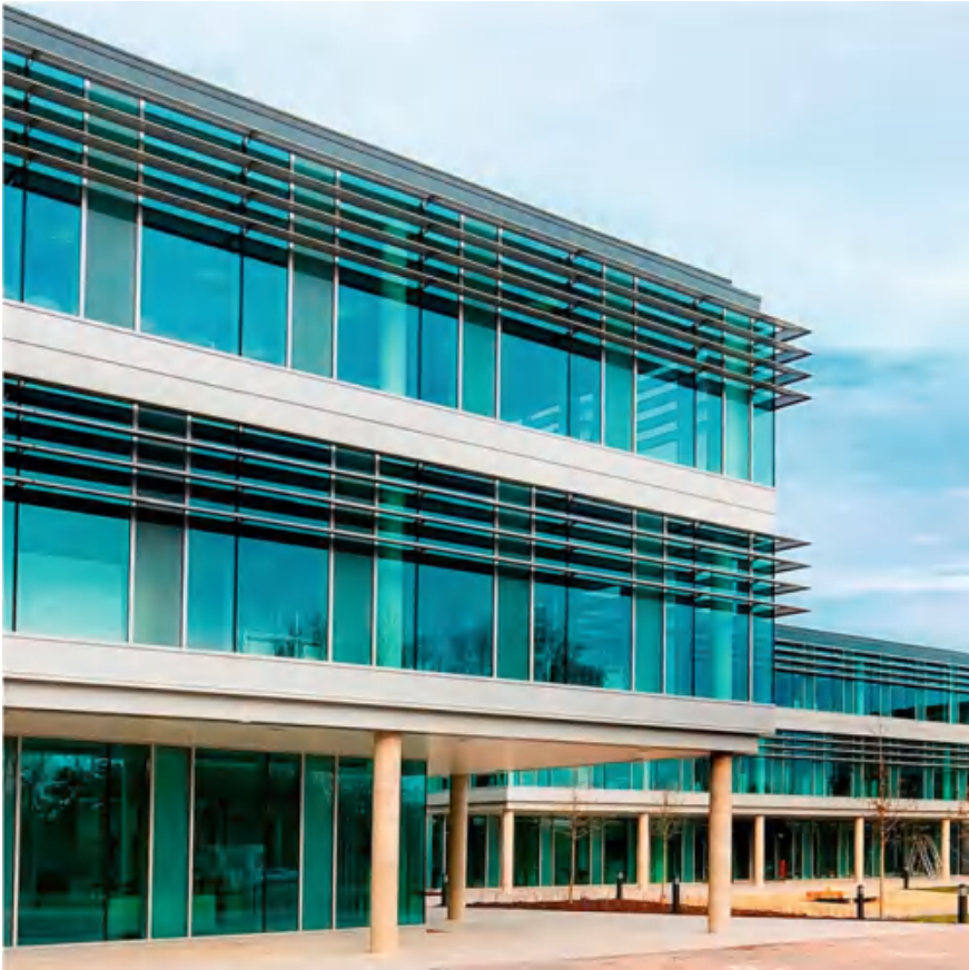
Fig. 4.6 Photo of a building with exterior horizontal shading fixtures (Levolux 2012)
