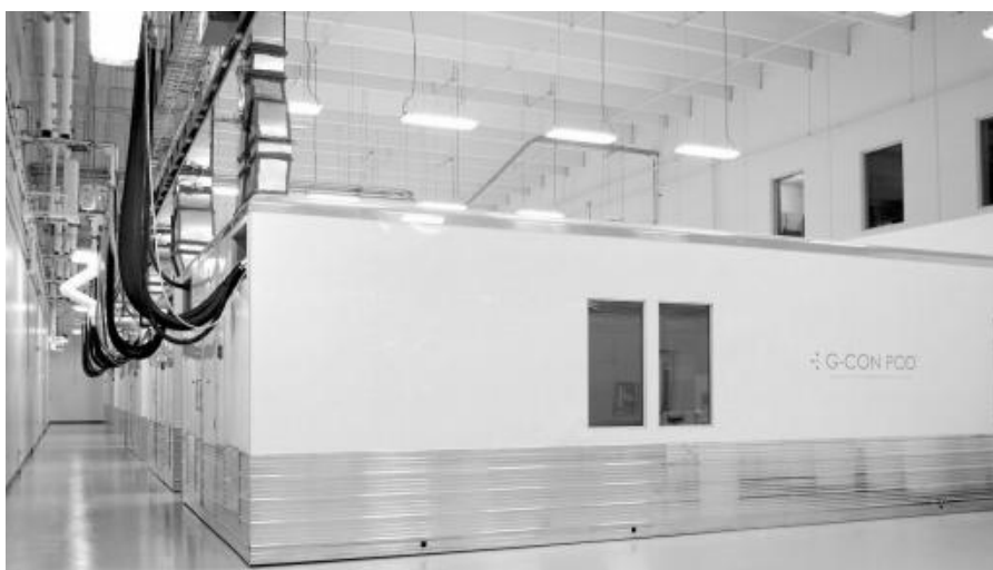
FIGURE 12.23 Prefabricated, autonomous clean room pod bioprocess. (Courtesy of G-CON Manufacturing, Inc., College Station, TX.)
