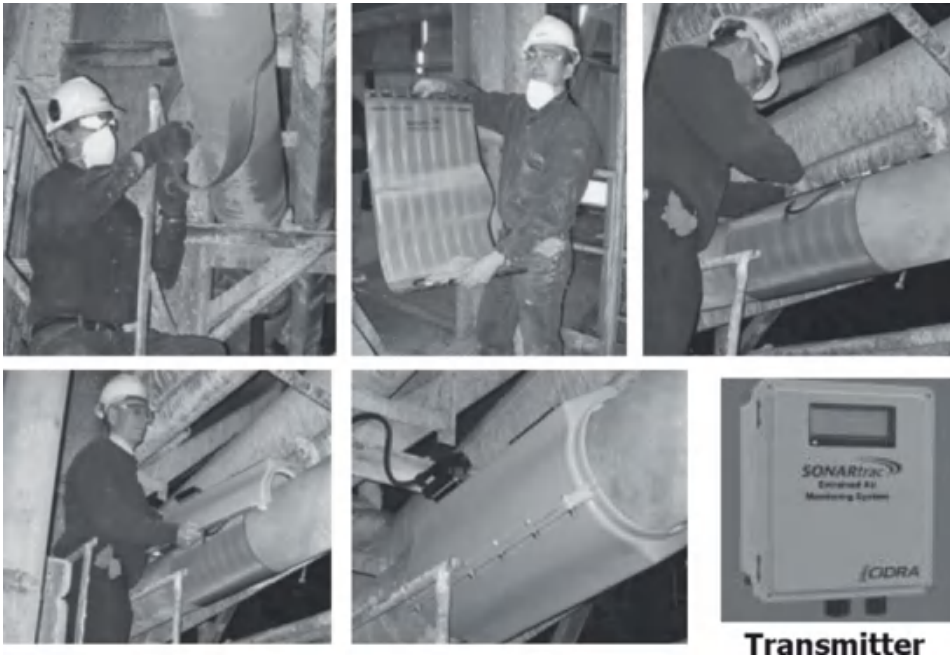
Figure 15.6. Installation procedure from (top-left) pipe preparation through cleaning and light sanding of pipe to (top-middle and top-right) mounting of the flexible, lightweight sensor band to (bottom-left) installation of the sensor cover and to (bottom-middle and bottom-right) connection of sensor cover to transmitter via watertight cable (reproduced with permission of CiDRA).
