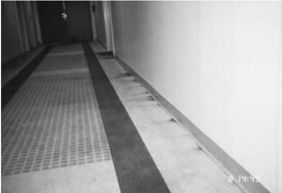
FIGURE 7.2 An Explosion is a Fire that Occurs in Milliseconds. Here Soot Was Deposited on the 97th Floor by the Supersonic Forces Generated.
