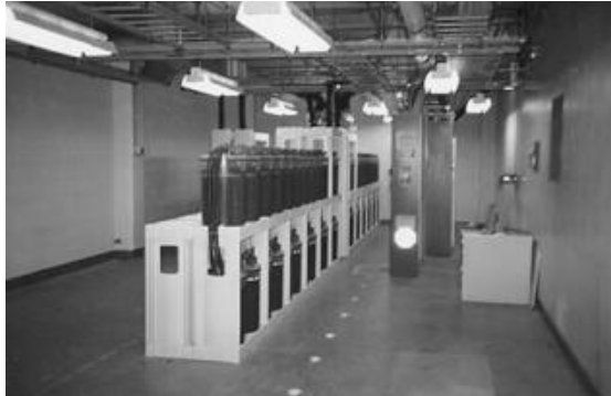
FIGURE 7.5 Batteries for UPSs and Office Power Should Be Isolated from the Rest of the Electronic Equipment to Prevent Corrosion from a Faulty Battery's Emissions.
