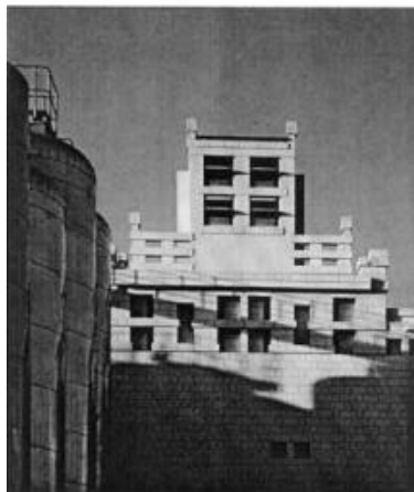
FIGURE 12.21 The Farsons Brewery in Malta by Short & Ford Eliminates the Need for a Refrigerant Cooling System by Using Wind Towers for Natural Ventilation. Top: Sectional Sketch; Bottom: Exterior View (Rickaby, 1991).
