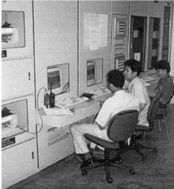
FIGURE 22.14 Honeywell Building Automation and Energy Management Systems—Bangkok Bank, Thailand.
