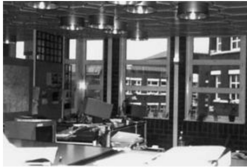
FIGURE 12.26 The Colonia Headquarters Has a Modular Reconfigurable Ceiling with Plug-and-Play Capability for Relocating Light Fixtures with Each Workstation Layout Change (ABSIC; Germany, 1989).
