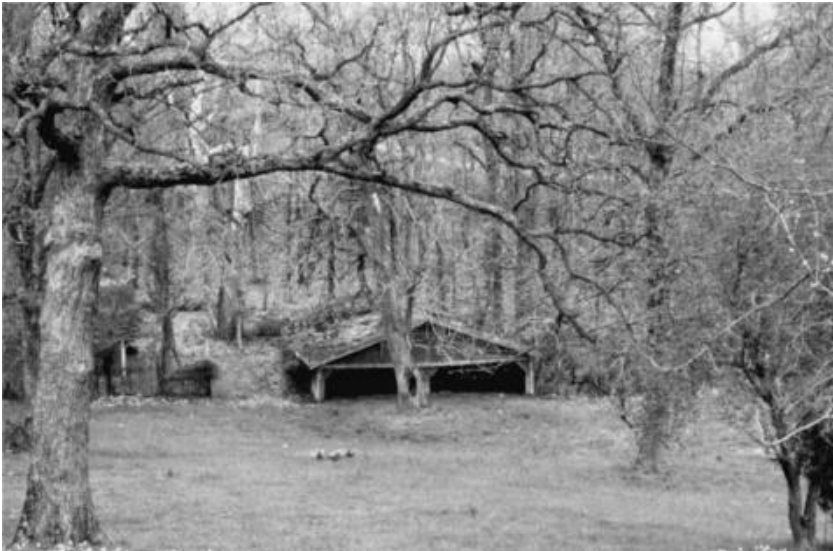
Figure 6.17. Barn located on floodplain along Drury Creek, southern Illinois. Floor has been buried by vertically accreted sediment produced by clear-cutting in the headwaters of the basin near the turn of the 20th century
