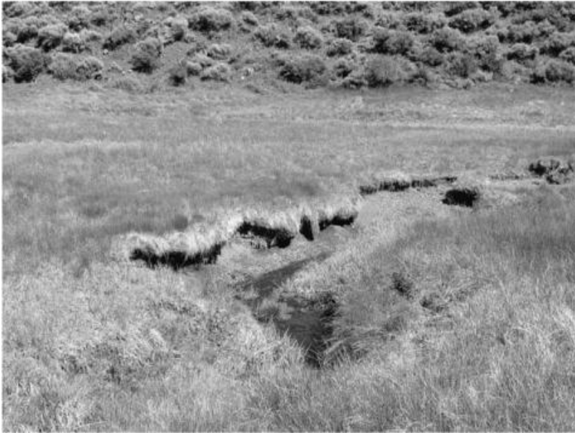
Figure 6.32. Corrasion of non-cohesive bank sediments, followed by failure of the overlying cohesive materials along Kingston Creek, Nevada
