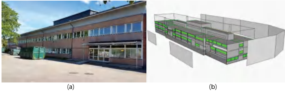
Figure 1. The school building, 97 m length, 18 m width, and 9 m height above the ground and the building energy simulation (BES) model, including shading objects such as trees shown in (a) and in (b) in form of screens.
