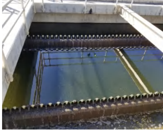
Figure 5.2: Sharp crested weir 27
