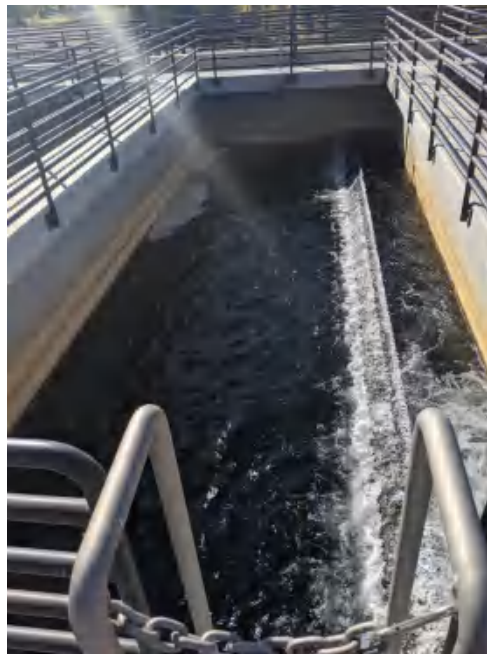
Figure 5.3: Broad crested weir 28
