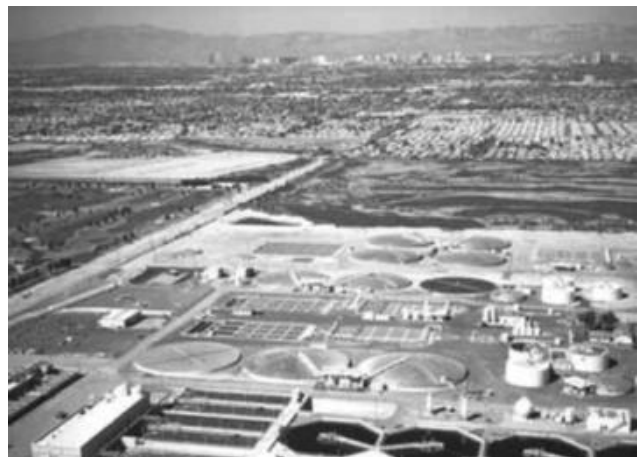
Figure 11.6 General view of a surface water treatment plant, http://www.epa.gov/waterinfrastructure/pdfs/brochure_si_sustainin_gounationswaters.pdf .
