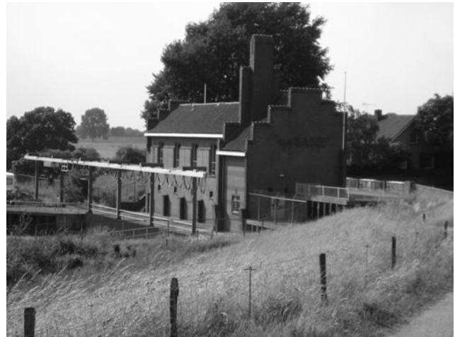
Figure 8.2 General view of the pumping station Van Sasse in Grave, the Netherlands (Source: http://en.wikipedia.org/wiki/Image:Gemaal_van_sasse.jpg ).
