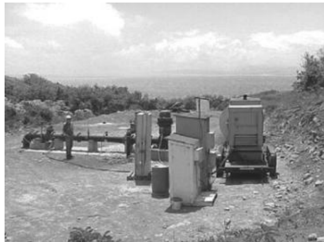
Figure 1.3 A well provides about 1.5 MGD (5.68 MLD) of water to Central Maui, HI (Courtesy of the Department of Water Supply, Maui County, HI).
