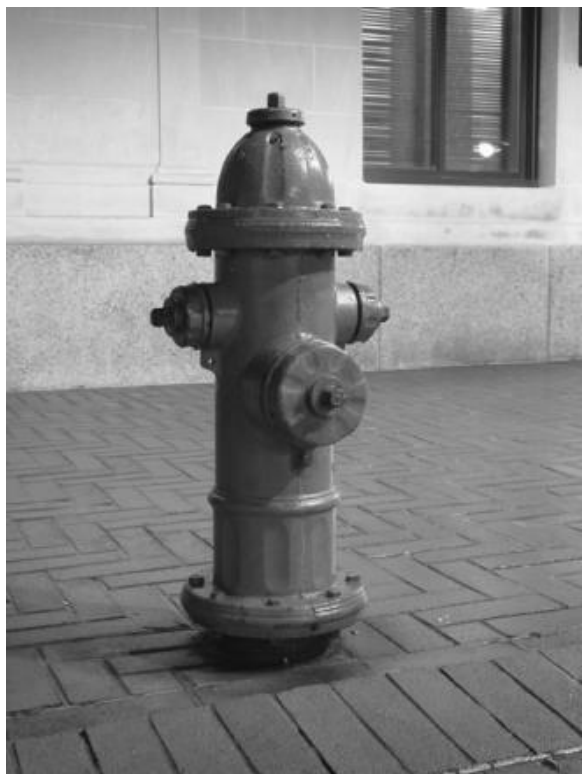
Figure 6.5 Fire hydrant (Source: http://en.wikipedia.org/wiki/Image:Downtown_Charlottesville_fire_hydrant.jpg ).
