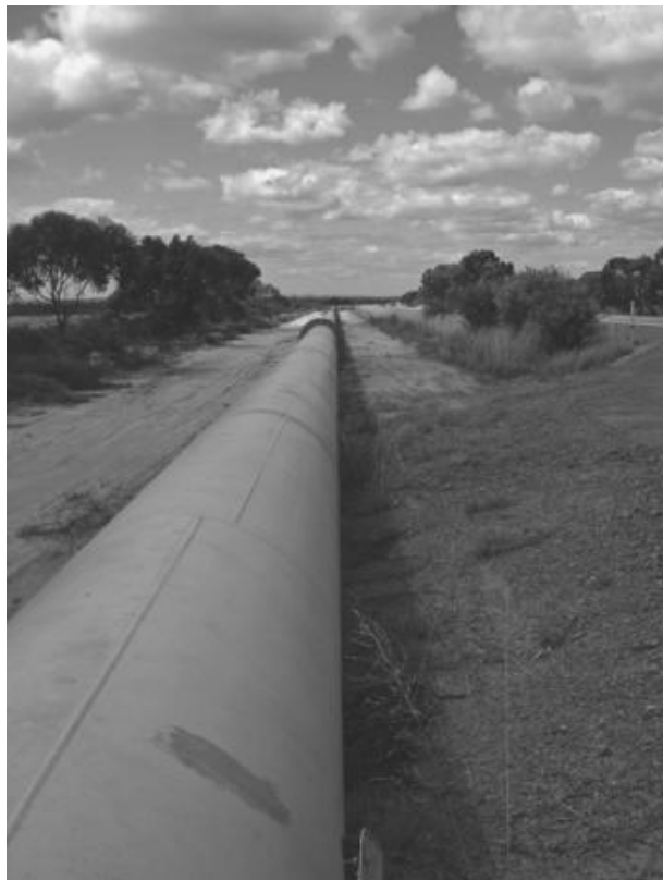
Figure 1.8 A pipeline in the Goldfields Water Supply Scheme, Perth, Australia (Source: http://en.wikipedia.org/wiki/Image:Goldfields_Pipeline_SMC.JPG ).
