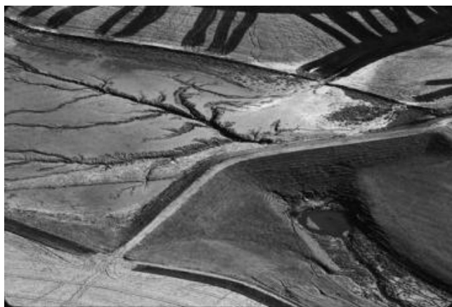
Figure 2.9 A watershed dam in northwest Iowa is completely silted in. The dam no longer functions to store water, since its capacity has been lost (Courtesy of the National Resources Conservation Service and USDA).
