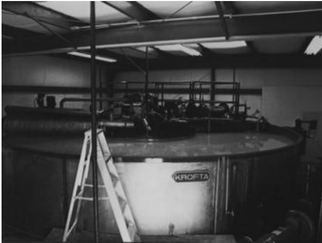
Figure 15.25 First US DAFF 1 MGD potable water treatment plant was built in 1982 in Lenox, MA (Krofta and Wang, 1985).
