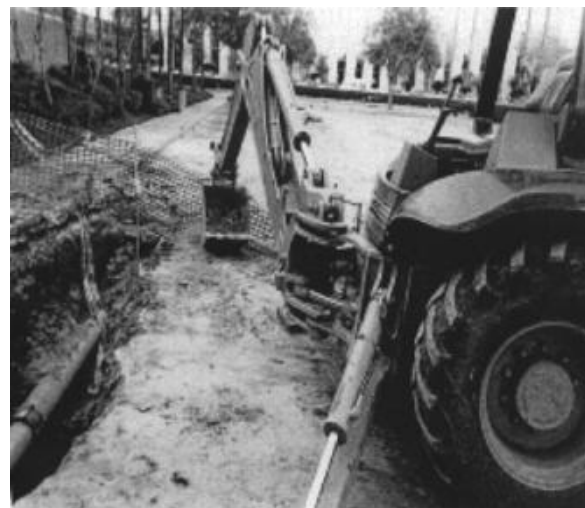
Figure 6.19 Bucket and boom of backhoe.
