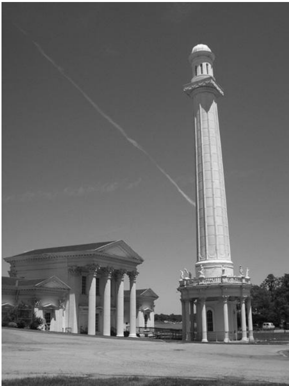
Figure 8.9 Water storage tank (Source: http://en.wikipedia.org/wiki/Image:Louisville_water_tower.jpg ).
