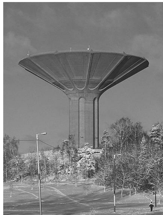
Figure 8.10 The mushroom-shaped concrete water tower in Helsinki, Finland. It is 52 m high and can hold 12,000 m 3 of water (Source: http://en.wikipedia.org/wiki/Water_supply_network ).
