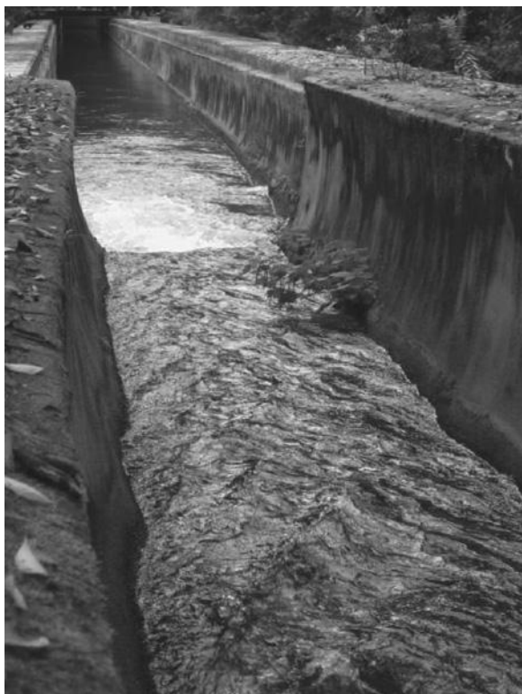
Figure 5.9 Water channel of the Nanzenji aqueduct, Kyoto, Japan (Source: http://en.wikipedia.org/wiki/Image:Nanzenji_aqueduct_channel.jpg ).
