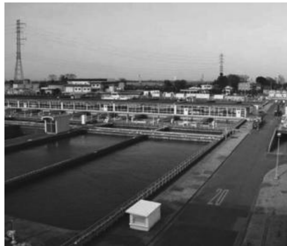
Figure 15.12 Rectangular sedimentation tanks (Courtesy of US EPA).
